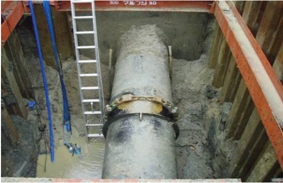
Photo 2 Excavation of joint failure portion.
