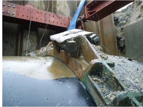
Photo 3 Sealing bolt worn out by hydro-blasting.
