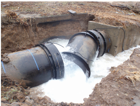
Photo 1 Water leakage from expansion joint.
