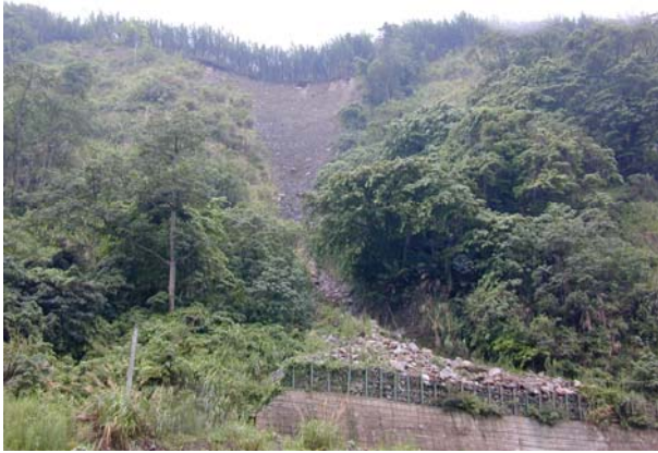
Fig. 6 HDF in Moi-Li after Chi-Chi earthquake.
