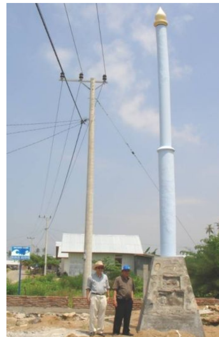
Figure 8. The Tallest Tsunami Pole Pole No.: 69, Height: 9.00 m (w), Distance from Shore: 0.50 km, Location: Masjid Lam Tengoh, Peukan Bada, Banda Aceh. The wave height was justified from witnesses, because there was no
