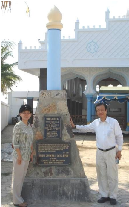
Figure 5. The Firstly Built Tsunami Pole (February 2006) Pole No.: 01, Height: 3.15 m, Distance from Shore: 2.80 km, Location: Gampong Lamdingin, Kecamatan Kuta Alam, Banda Aceh. The placard in front of the pole shows the inundation height, distance from shore, time of tsunami arrival, time of earthquake, location name, words of wisdom, developer, and donor
