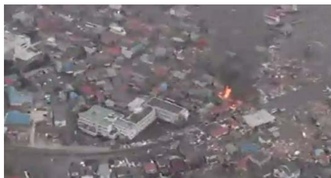
Fig. 29 Fire situation at 16:15 11 th March 2011 about one hour after the tsunami hit here Yamada district in Yamada town (JGSDF, 2011)
