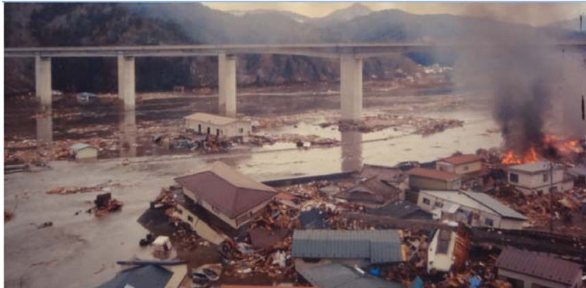
Fig. 13 Fire spread at Origasa district at 16:07 of 11 th March 2011 ( photograph taken and offered by local people )
