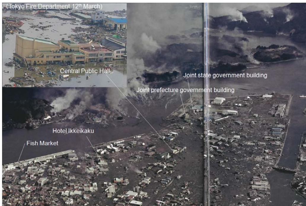
Fig. 38 Tsunami Evacuation Buildings at Harbor district in Kesenuma (Bon Ishikawa, 2011)
