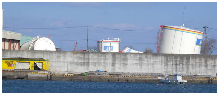
Fig. 7 Oil tanks damaged in the Port of Kuji
