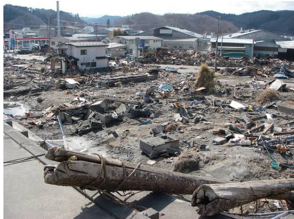
Fig. 13 Destruction of residential area behind a protection dike
