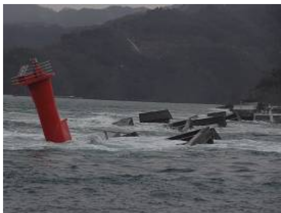
Fig. 10 North offshore breakwater damaged in the Port of Kamaishi
