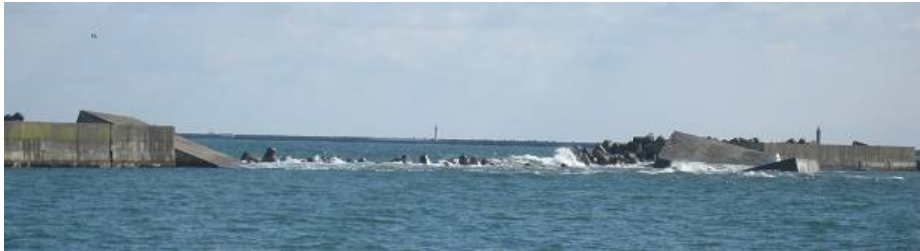
Fig. 5 Breakwater damaged in the Port of Hachinohe
