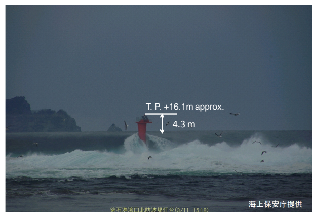
Fig. 11 Tsunami overtopping the north offshore breakwater in the Port of Kamaishi (Photo courtesy of Japan Coast Guard)
