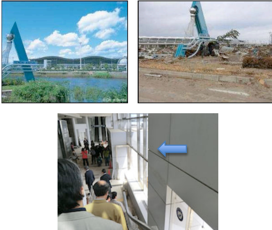
Photo 2 Sendai international airport before and after the 2011. The first floor was inundated c Ports causing serious damage on the operation system
