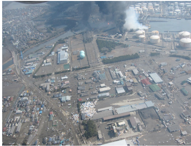
Photo 5 Damage due to the tsunami followed by fires at Sendai port
