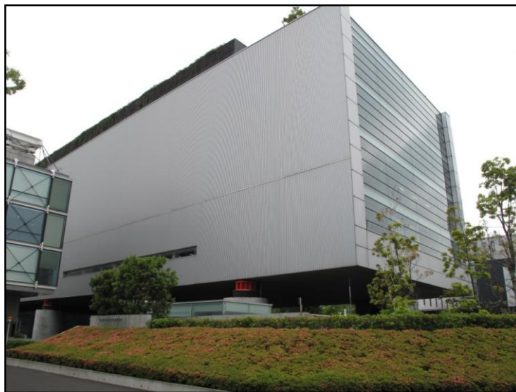
Fig. 9 Main Building at the Shimizu Institute of Technology
