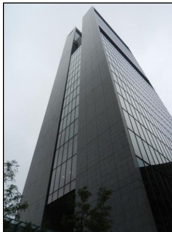
Fig. 7 Yozemi Tower, in the Shinjuku area of Tokyo
