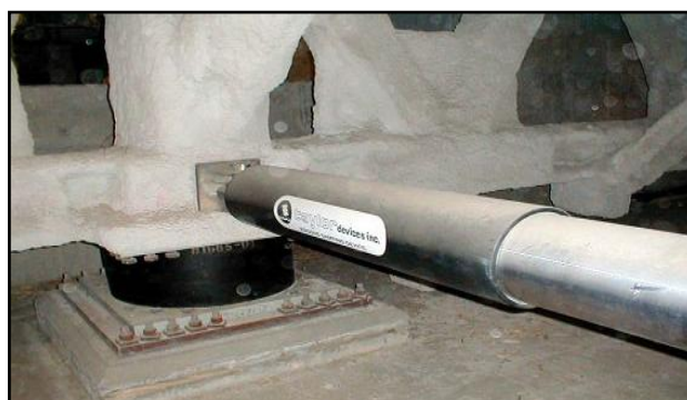
Fig. 1 Oil damper in combination with high damping rubber seismic isolation bearings, Arrowhead Regional Medical Center, San Bernardino County, California
