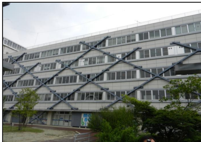
Fig. 3 Exterior steel frame for seismic strengthening of Building B5 at Tohoku Institute of Technology
