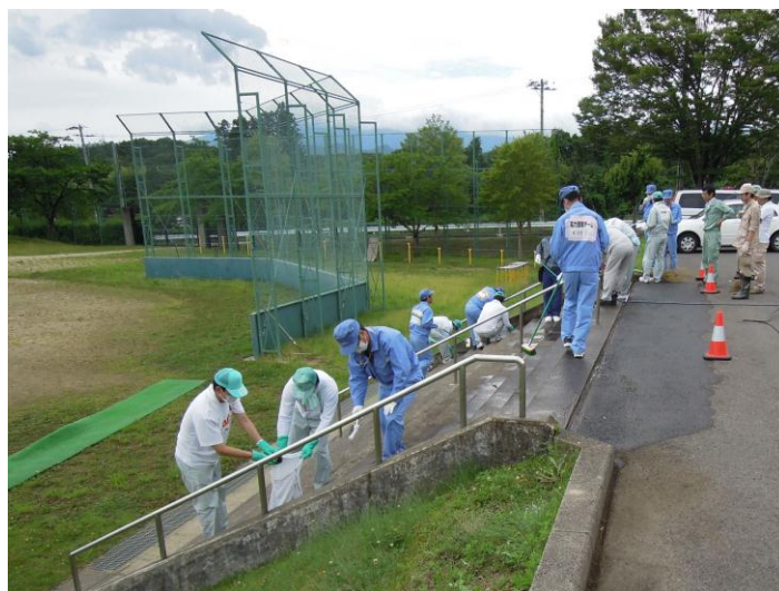
Photo 1. Decontamination work at an elementary school (Fukushima City, June 2011).
