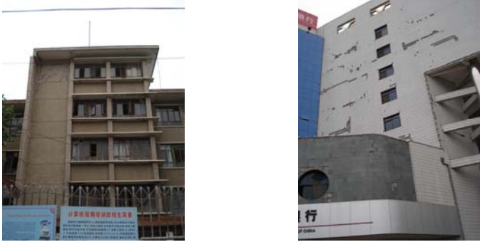
(a) Irregular building in planar direction (b) Irregular building in planar direction and façade
