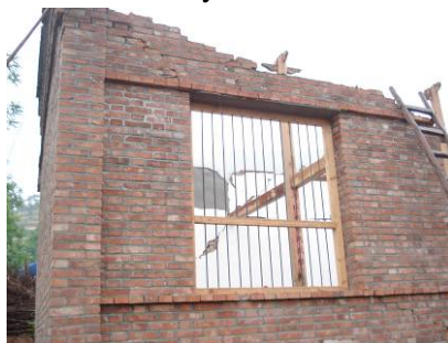
Fig.4 The destroyed masonry timber buildings
