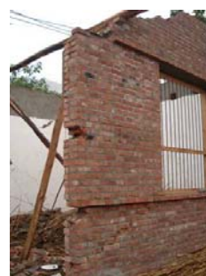
Fig.4 The destroyed masonry timber buildings
