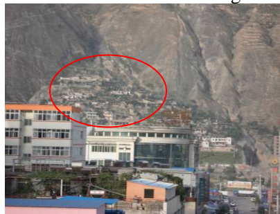
Fig.11 The buildings built on landslide zone
