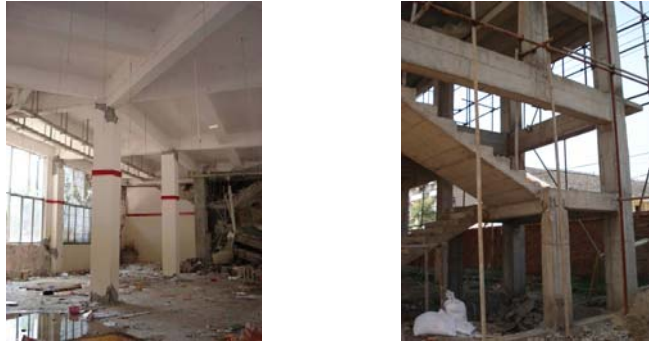
Fig.8 The phenomenon of ‘strong beam-weak column’
