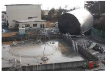
Photo 5 Fuel tank floated and dislocated (by Tohoku EPCO)
