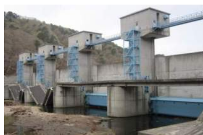
Photo 3 Tsunami wall across Fudai River (Fudai, Iwate Prefecture)
