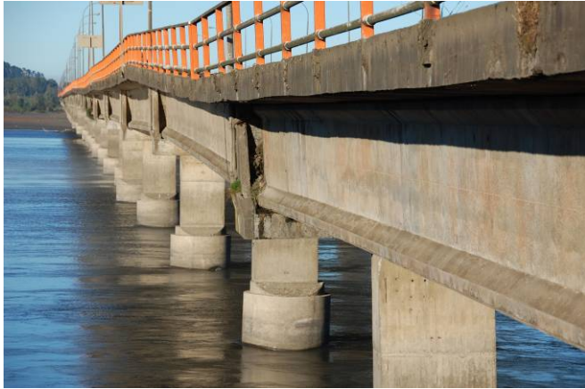
Photo 14 Damage of Juan Pablo II Bridge (Left: Settlement of Pier Foundation, Right: Shear Failure of Pier Columns)
