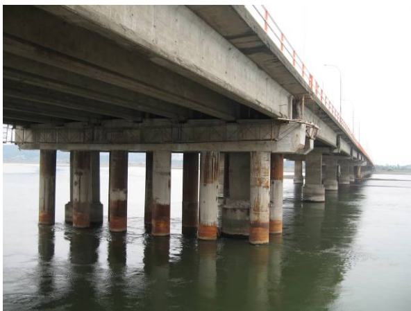
Photo 15 Repair and Retrofit of Juan Pablo II Bridge (Left: Additional Piles at settled Piers, Right: Replaced Pier Columns and Lateral Stopper Structures)
