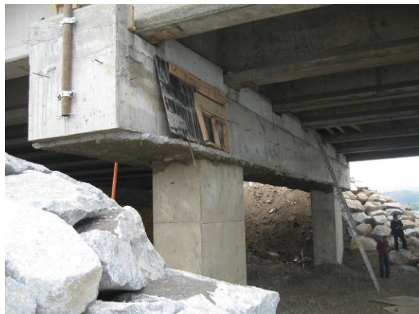
Photo 15 Repair and Retrofit of Juan Pablo II Bridge (Left: Additional Piles at settled Piers, Right: Replaced Pier Columns and Lateral Stopper Structures)
