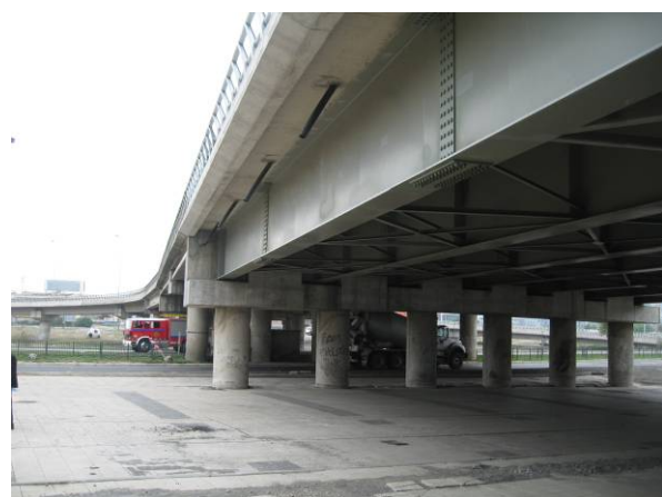
Photo 17 Replaced Collapsed Span of Llacolen Bridge
