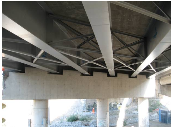
Photo 13 Reconstruction and Retrofit of Hospital Overpass (Left: Side View, Right: Lateral Stopper at Cap Beam of Pier)
