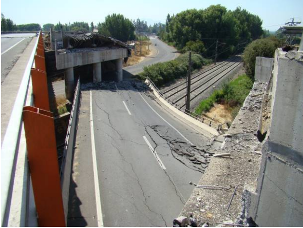
Photo 12 Collapse of Spans at Hospital Overpass
