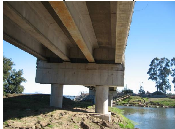
Photo 20 Lateral Displacement of Superstructure and Foundations at La Mochita Bridge
