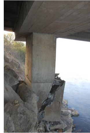
Photo 14 Damage of Juan Pablo II Bridge (Left: Settlement of Pier Foundation, Right: Shear Failure of Pier Columns)
