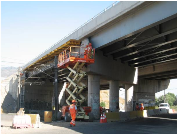
Photo 13 Reconstruction and Retrofit of Hospital Overpass (Left: Side View, Right: Lateral Stopper at Cap Beam of Pier)
