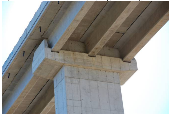
Photo 2 Bridges designed by Original Chilean Practice with End Diaphragms and Lateral Stopper Mechanism
