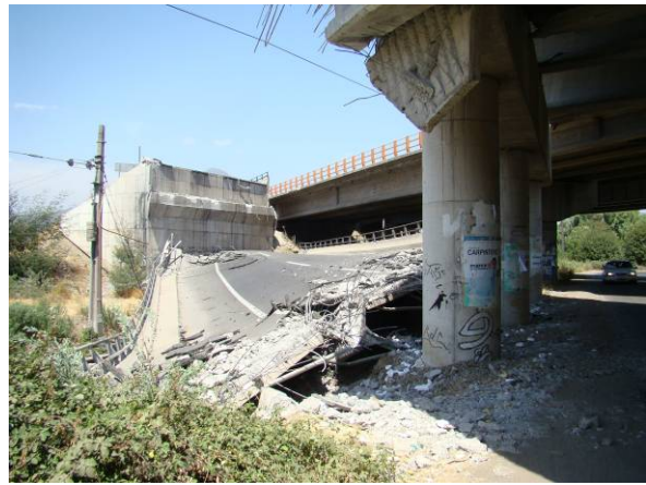
Photo 12 Collapse of Spans at Hospital Overpass
