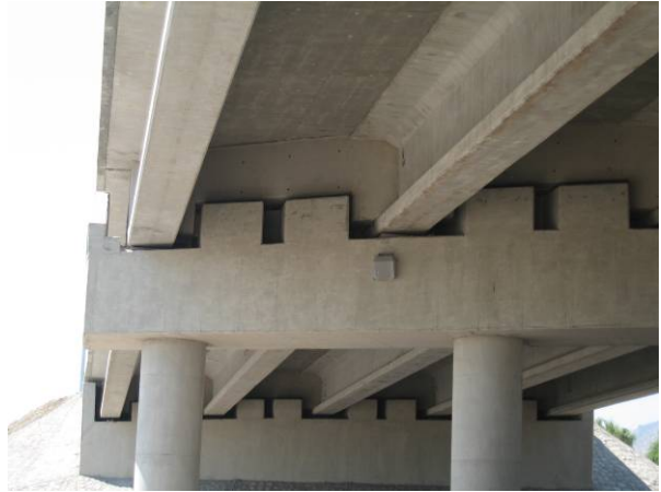
Photo 10 Repair and Retrofit for Los Pinos Bridge (Left: Side View, Right: Lateral Beams and Lateral Stoppers at Pier Cap)
