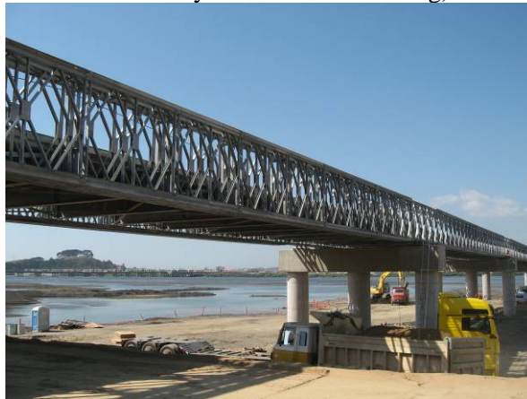
Photo 19 New Bridge Construction (Chacabuco Bridge) to cross BioBio River
