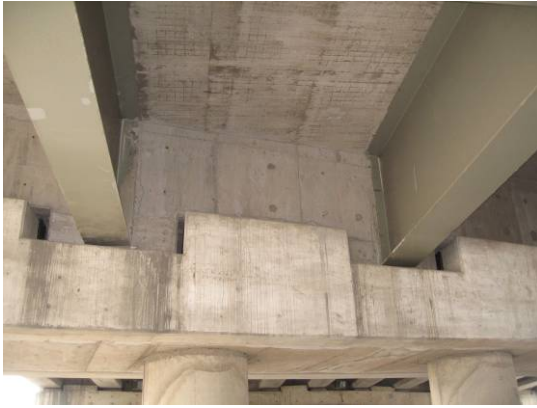
Photo 18 Repair and Retrofit for Llacolen Bridge (Left: Placement of Lateral Beams and Lateral Stoppers, Right: Widening of Pier Cap and Retrofitted Column by Fiber-Sheet Jacketing)
