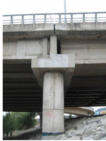
Photo 18 Repair and Retrofit for Llacolen Bridge (Left: Placement of Lateral Beams and Lateral Stoppers, Right: Widening of Pier Cap and Retrofitted Column by Fiber-Sheet Jacketing)
