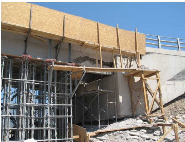
Photo 11 Repair and Retrofit for Azufradero Bridge (Left: Damage to Girders and Abutment, Right: Stiffening Wall at Backside of Abutment)
