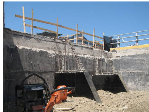
Photo 11 Repair and Retrofit for Azufradero Bridge (Left: Damage to Girders and Abutment, Right: Stiffening Wall at Backside of Abutment)
