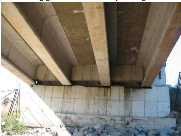
Photo 20 Lateral Displacement of Superstructure and Foundations at La Mochita Bridge
