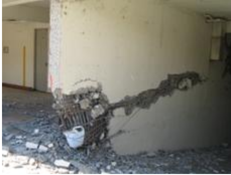
Fig. 11 Building B, Concepcion: Compression, tension and shear failure on first and second floors
