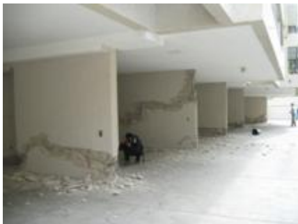
Fig. 12 Building C, Viña del Mar: general wall failure at first floor: 40 cm out of plumb at the top.
