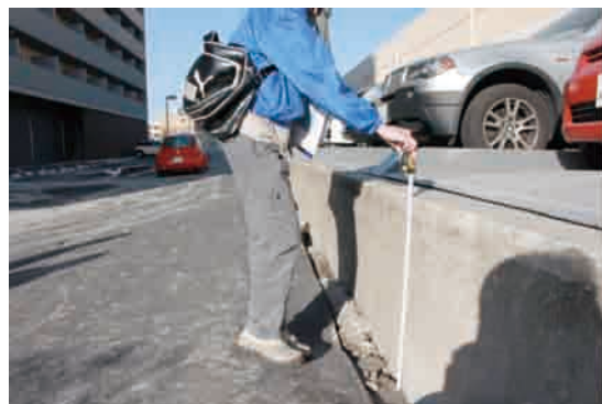
Photo 6 Uplifted underground parking garage 4)
