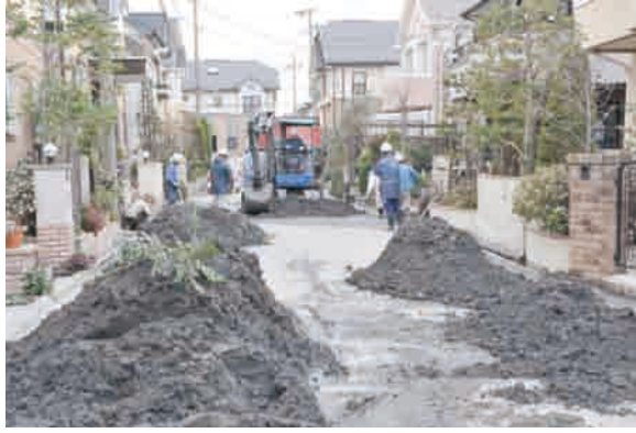
Photo 1 Sand boils stacked over the road
