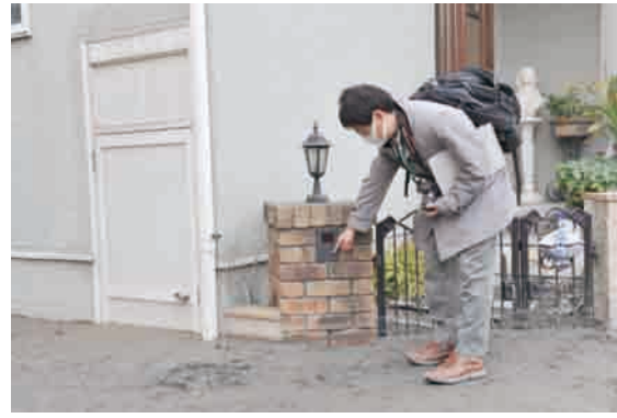
Photo 2 Wooden house suffering large settlement
