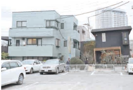
Photo 3 Buildings suffering large settlement and tilting 4)
