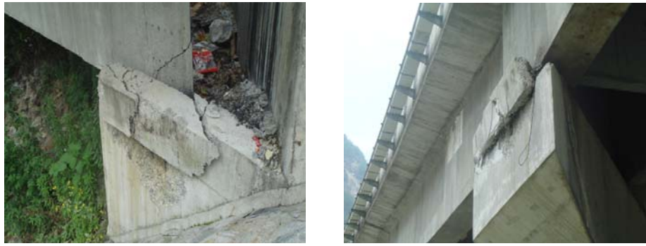
a Abutment 0 b . Bent 1 Fig. 5 Failure of shear keys of Duxiufeng Bridge
