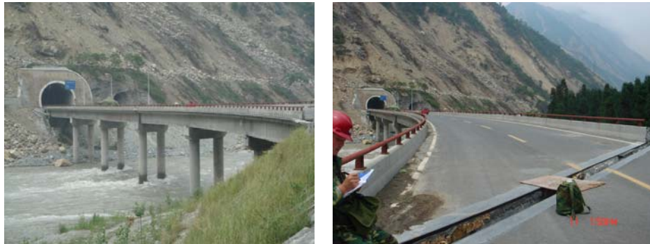
Fig. 2 Overview of Duxiufeng Bridge after the earthquake
