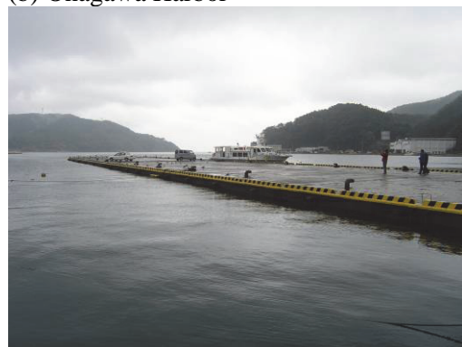
Fig. 4 Inundation and low ground level caused by coseismic subsidence (in Miyagi Prefecture)
