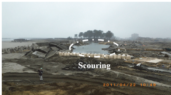
Fig. 1 Destroyed shape of sea wall near the mouth of Abukuma River
