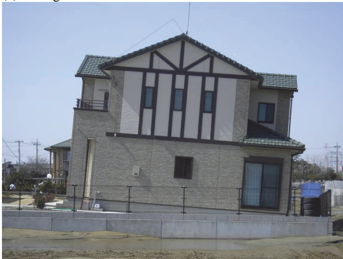
Fig. 11 Damage of private houses caused by liquefaction
