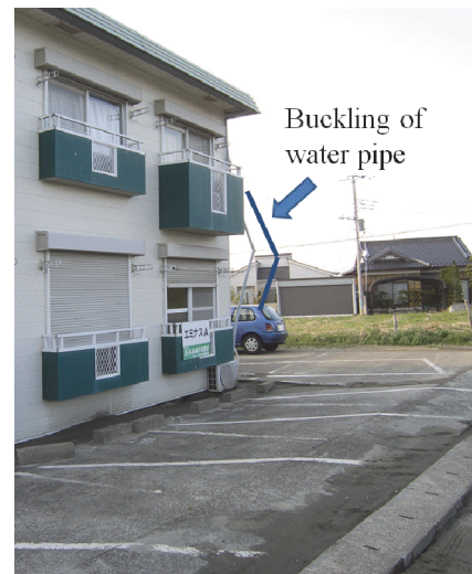
Fig. 11 Damage of private houses caused by liquefaction
