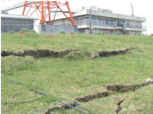
Fig. 6 Damaged levee of Tone River in Sawara
