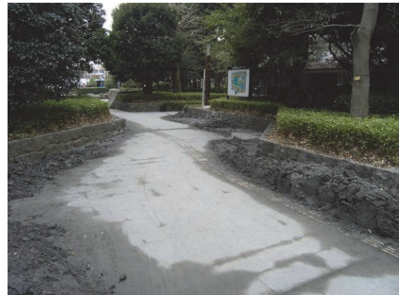
Fig. 12 Contrast of liquefaction in manmade island of Urayasu City
