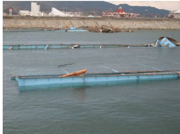
Photo 7 Damage of Kesen Bridge (2) (Left: Distance of Washed-out Superstructure, Right: Deformed Steel Girders)
