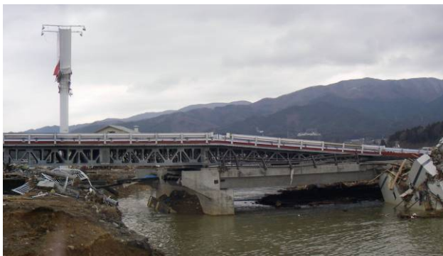
Photo 14 Emergency Recovery for Kawaharagawa Bridge (Left: Construction of Temporary Girders (Tohoku Bureau of MLIT, 2011c), Right: Refilled Backfill of Scoured Abutment)
