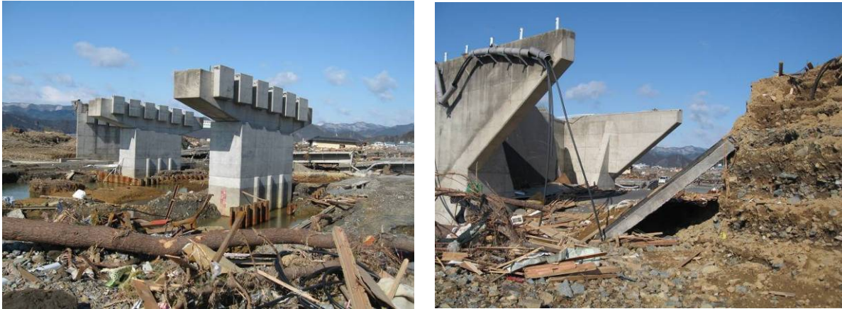
Photo 11 Damage of Numata Bridge (Left: Survived Piers, Right: Heavy Scouring of Backfill Soil at Abutment)
