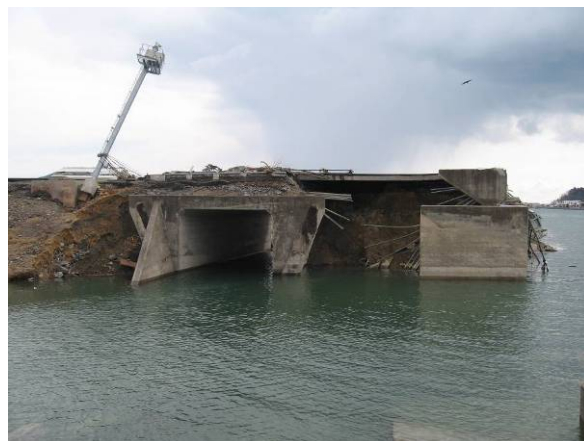
Photo 8 Scouring of Abutment Backfill of Kesen Bridge
