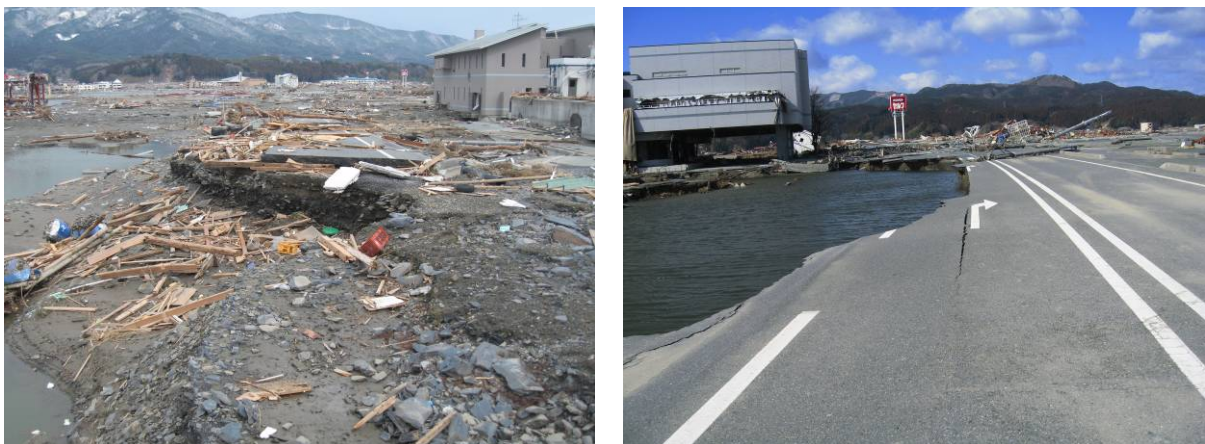
Photo 5 Peeling-off of Road Pavement and Scouring of Soil Sections
