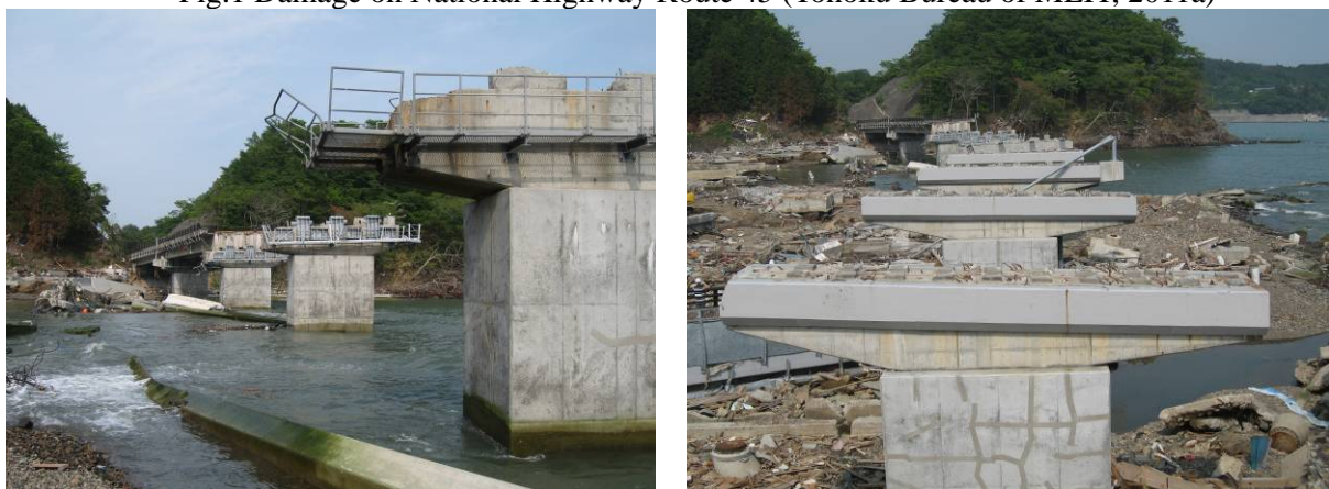
Photo 1 Typical Heavy Damage of Bridges: Wash-out of Superstructures by Tsunami
