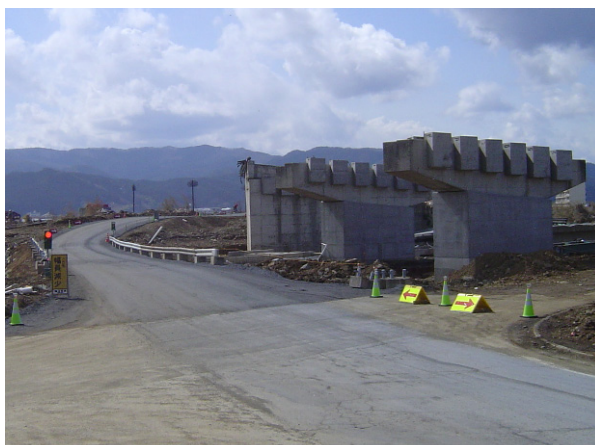
Photo 11 Construction of Temporary Road beside Numata Bridge (Tohoku Bureau of MLIT, 2011c)
