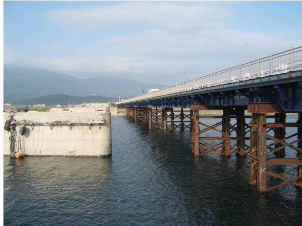
Photo 13 Construction of Temporary Bridge at Kesen Bridge
