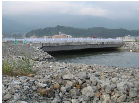
Photo 14 Emergency Recovery for Kawaharagawa Bridge (Left: Construction of Temporary Girders (Tohoku Bureau of MLIT, 2011c), Right: Refilled Backfill of Scoured Abutment)
