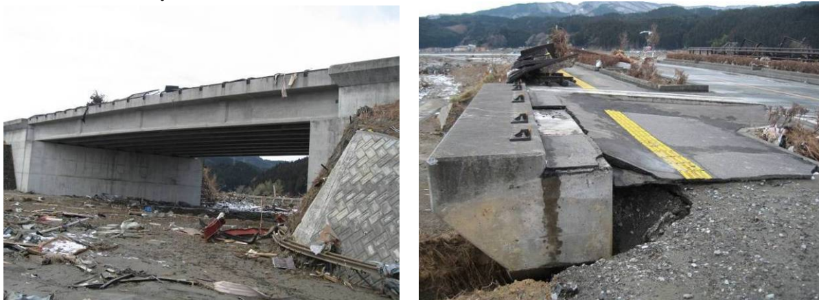
Photo 12 Investigation of Nanakiri Bridge (Left: Side View, Right: Slight Scouring of Backfill Soil at Abutment)
