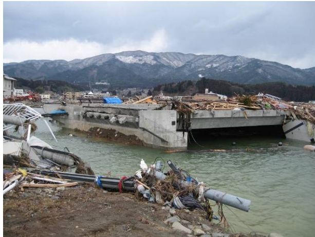
Photo 9 Wash-out of Backfill Soil of Kawaharagawa Bridge
