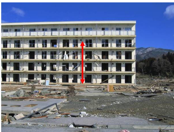
Photo 2 Tsunami Height in Rikuzen-Takada City: Around 10m
