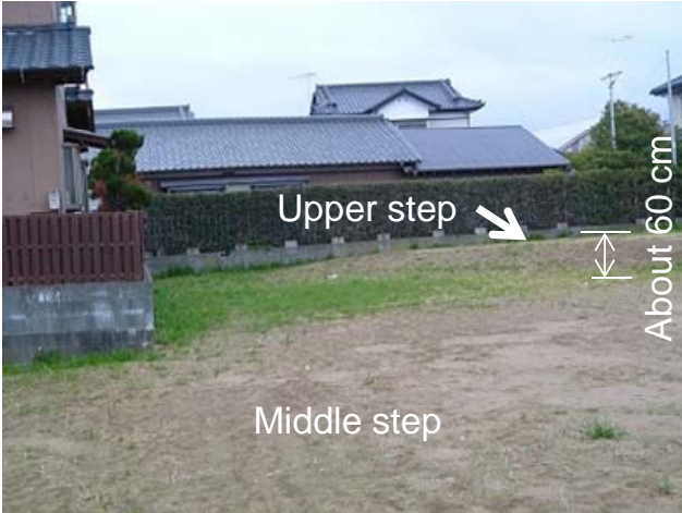
Photo 5 Up-heaved field due to liquefaction of soil
