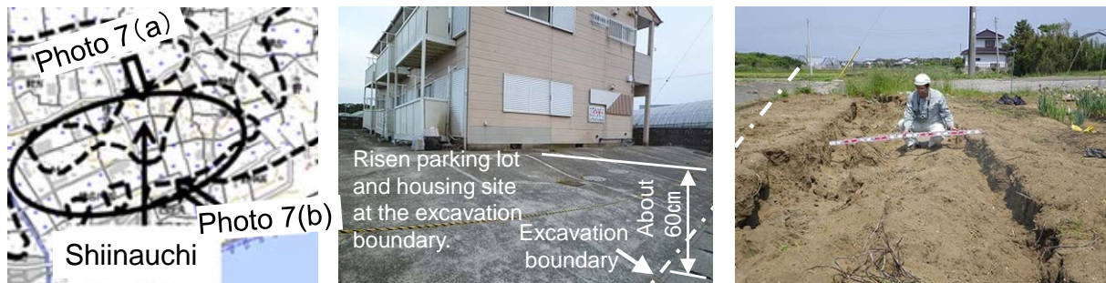
(a) Upheaval at north boundary (b) Cave-in at south boundary
