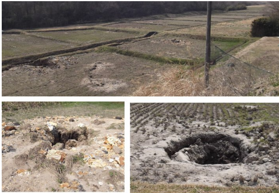
Fig. 10 Views of sinkholes in a rice field near Ohira Village
