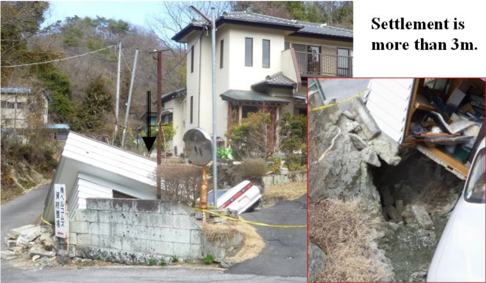
Fig. 19 The settlement of back-filling material of the shaft and the fall of the hut and car into the shaft
