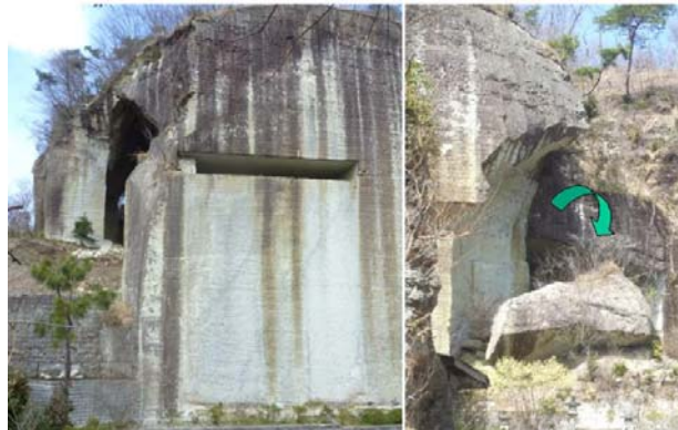
Fig. 17 Partially collapsed semi-underground opening
