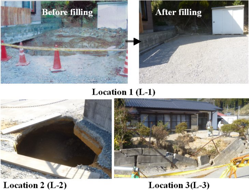
Fig. 6 Views of sinkholes locations L1-L3
