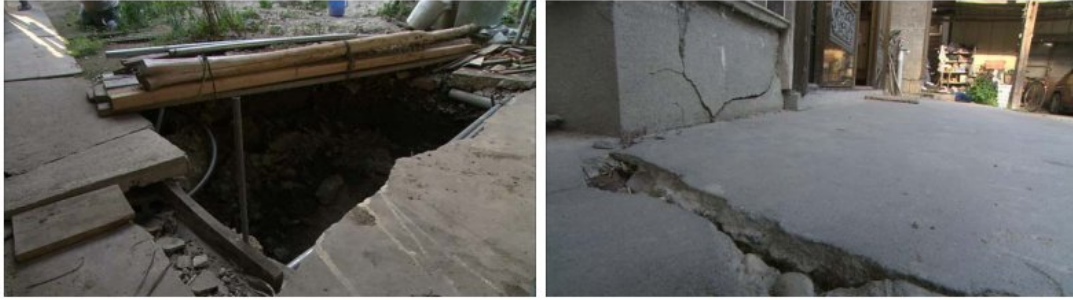
Fig. 13. A sinkhole beneath a house in Ichinoseki. (L2)
