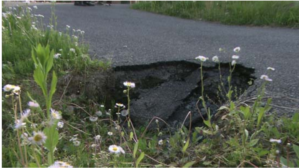
Fig. 14 Sinkhole beneath the roadway in Ichinoseki (L3)
