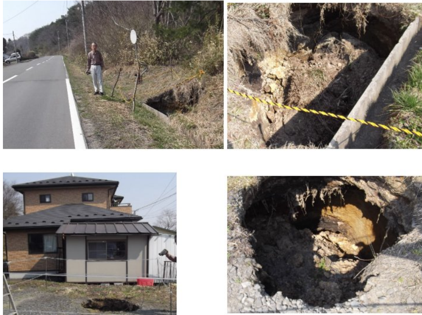
Fig. 11 Views of sinkholes along a roadway and parking lot near Ohira Village
