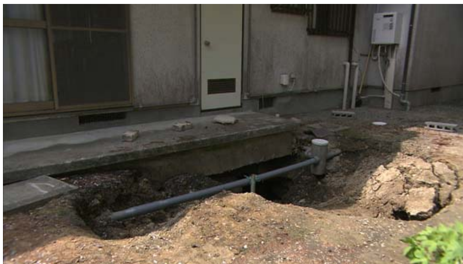
Fig. 12 A sinkhole beneath a house in Ichinoseki. (L1). The size of the sinkhole enlarged after the April 7, 2011 aftershock
