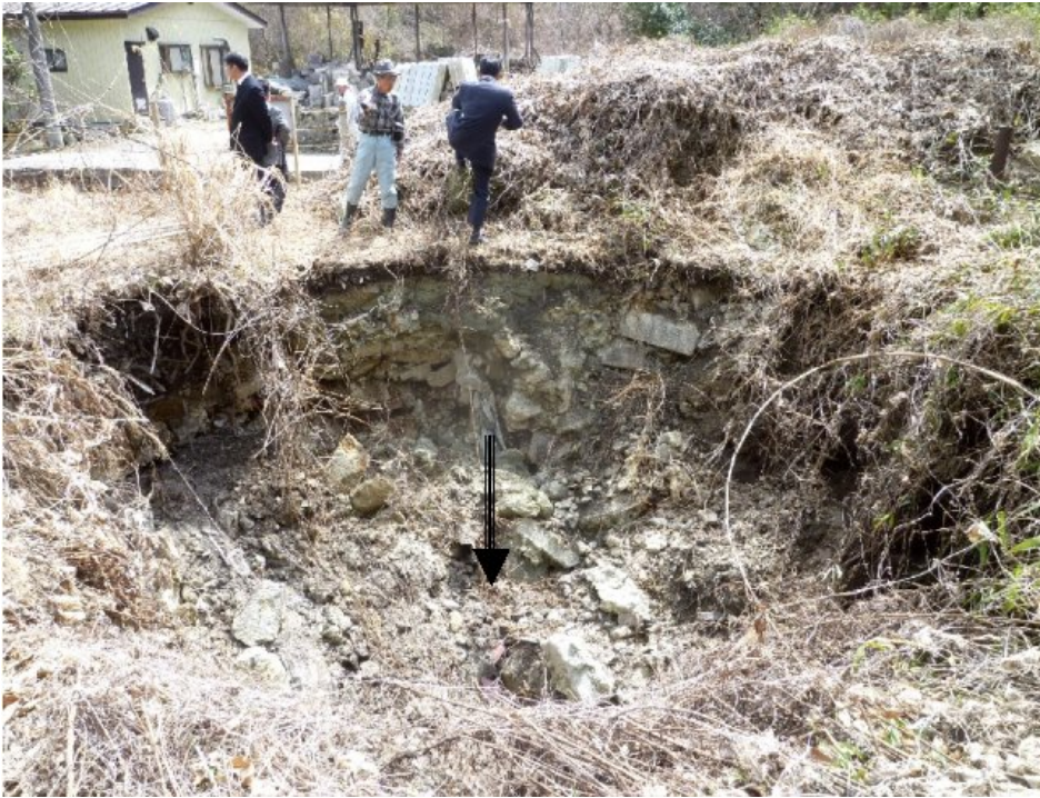
Fig. 18 The settlement of back-filling material of the shaft
