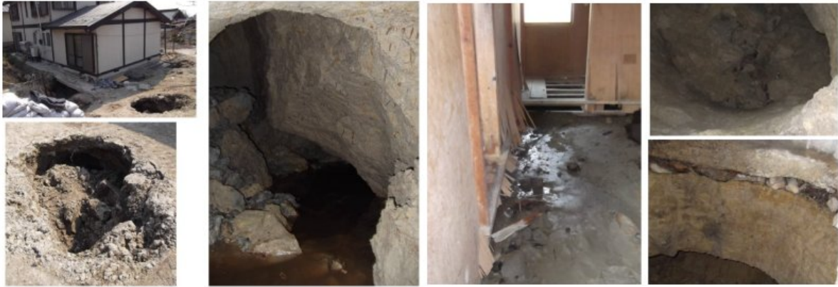
Fig. 9 Views of sinkholes and related damage in Wakayanagi town
