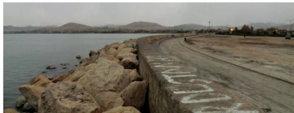
(c) Liquefaction and lateral spreading at Van Port (Van lake shore)
