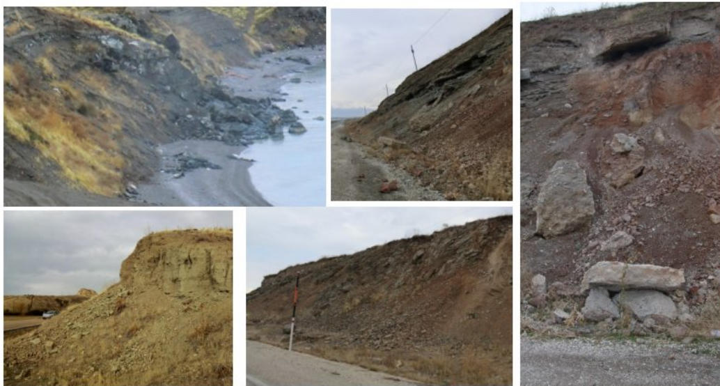
Photo 4 Rock slope failures at several localities
