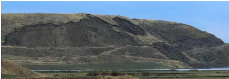
Photo 3 Slope failure near Topraktaş
