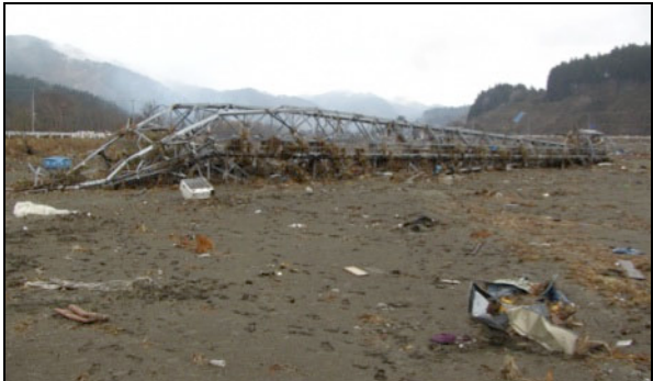
Figure 15. Cell site destroyed by the tsunami in Rikuzentakata
