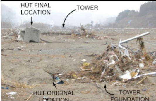
Figure 15. Cell site destroyed by the tsunami in Rikuzentakata
