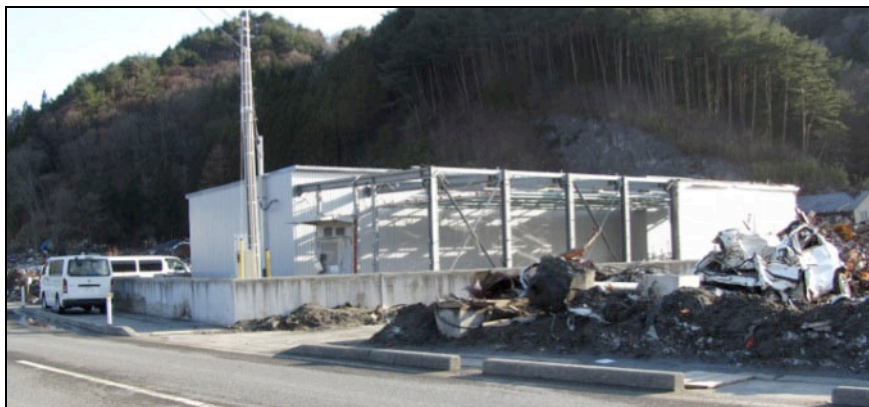
Figure 12 Unosomai CO, side and roof were replaced on the back half of the building
