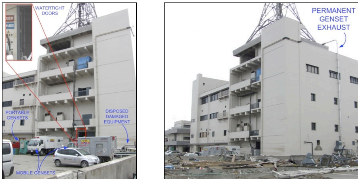
Fig. 2 Ofunato CO with more than one mobile power generators
