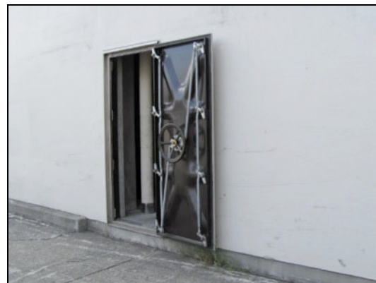
Figure 5. Left: A portable genset at Kamaishi CO with a truck of additional diesel storage expecting very long autonomies. Right: Watertight door at Kamaishi CO.
