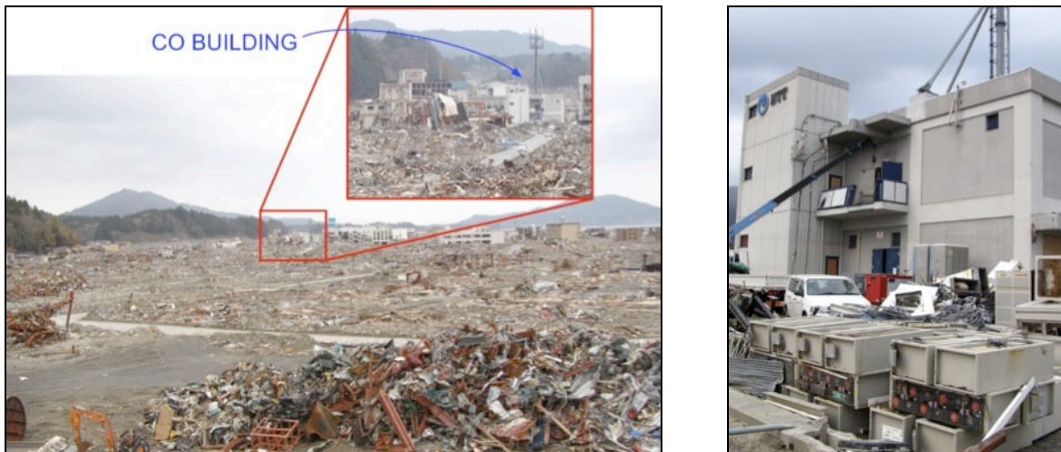
Figure 11 Rikuzentakata CO. Right: Disposed water damaged batteries.
