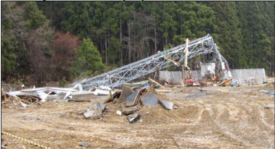
Figure 16. A collapsed tower of a base station located in the Karakuwa Peninsula.
