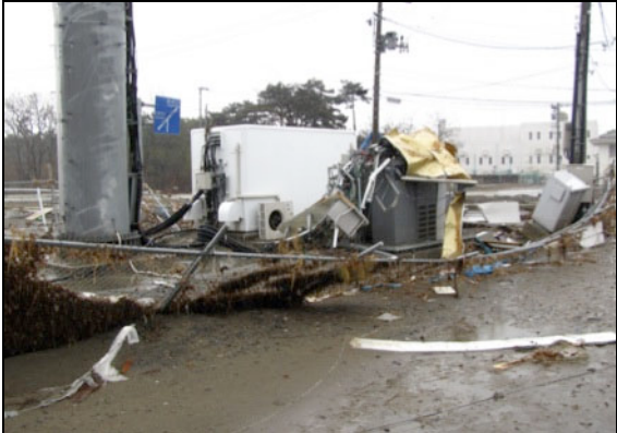
Figure 14. Destroyed cell site at Ishinomaki
