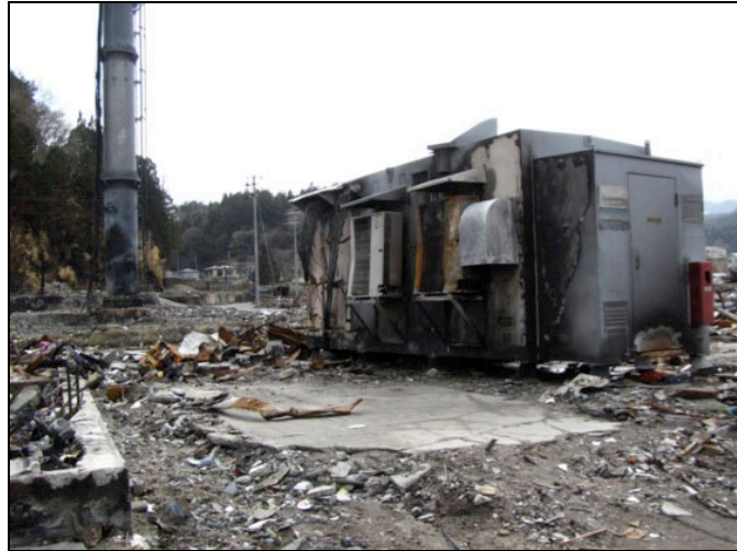
Figure 17. This base station in Yamada was also damaged by fire in addition to tsunami damage
