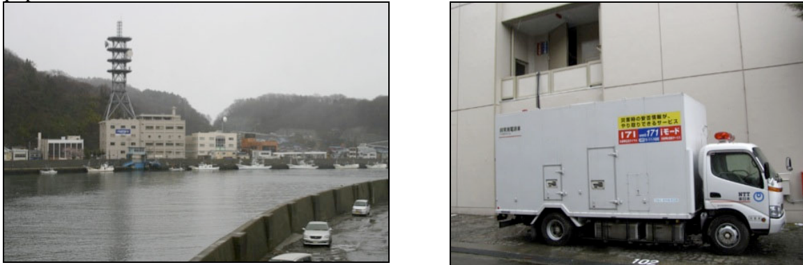
Fig. 1 Miyako CO on the left and the mobile power generator on the right
