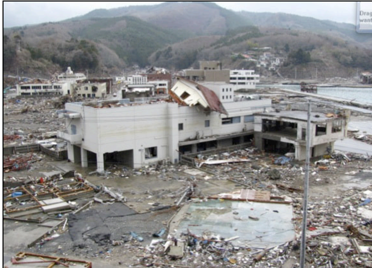
Figure 10. Onagawa CO with a roof of another house on its roof.
