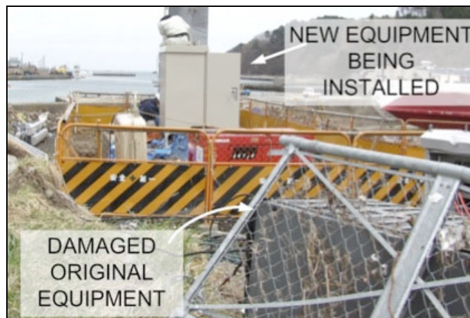
Figure 20. New base station equipment was being installed in Heita.
