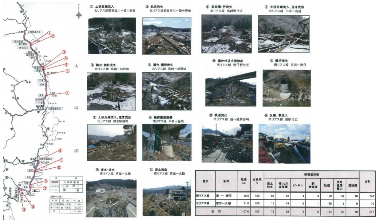
Fig. 8 details and place of damage
