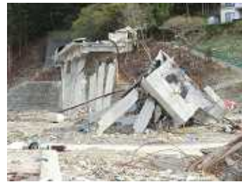
Fig.10 Washout of Shimanokoshi Sta.
