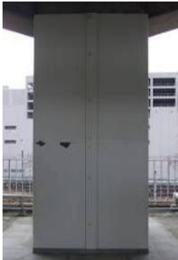
Photo 2 Impact by earthquakes on columns with seismic rehabilitation by Steel plate jacketing method using indented joints
