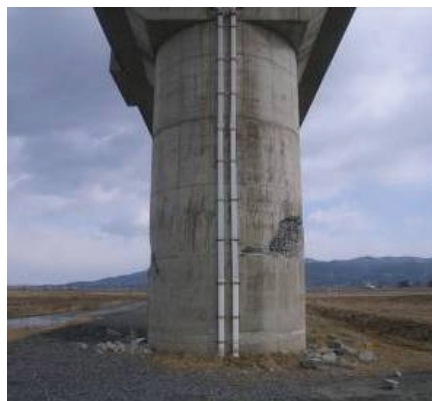
Photo 5 Example of seismic damage of RC bridge piers (damage level B)
