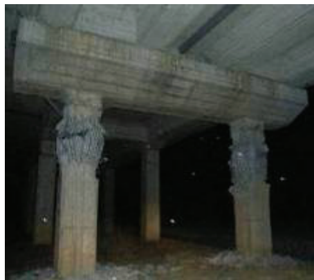
Photo 1 Example of seismic damage of RC viaduct columns (damage level BB)
