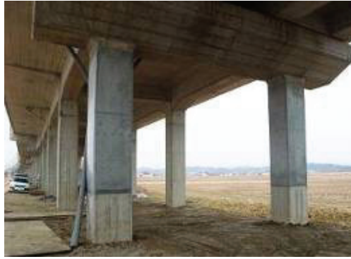
Photo 6 Restored RC columns
