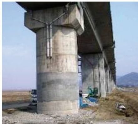
Photo 7 Restored RC pier
