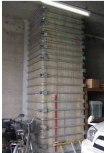
Photo 3 Impact by earthquakes on columns with seismic rehabilitation by Rib-Bar method
