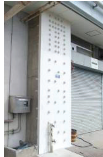
Photo 4 Impact by earthquakes on columns with seismic rehabilitation by Single-face method
