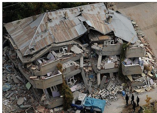
Fig 9. Damaged Reinforced Concrete buildings in Erciş (AA Press)
