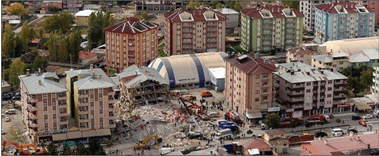
Fig 7. Damaged Reinforced Concrete buildings in Erciş (AA Press)
