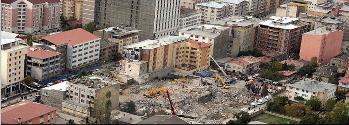
Fig 10. Damaged Reinforced Concrete buildings in Van (AA Press)
