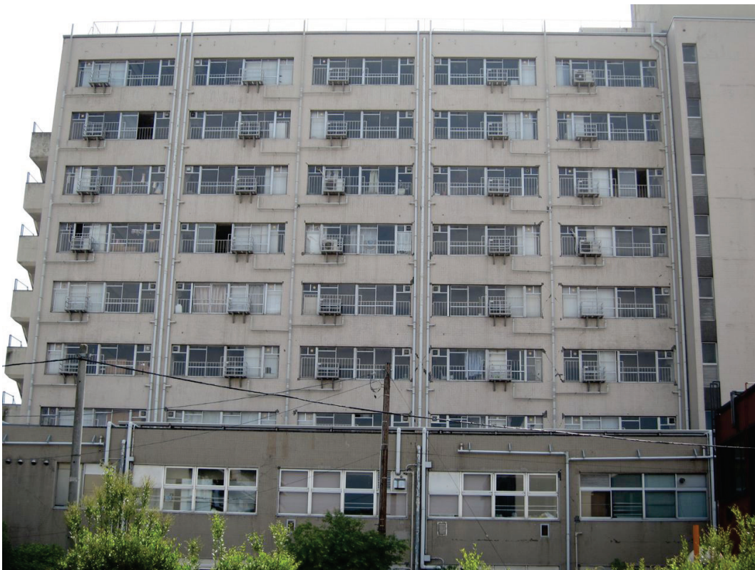
Fig. 1 Overview of the N-Building from the west side
