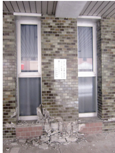
Fig. 7 Column X_1-Y_1 at 1st floor with concrete crushing and rebar buckling
