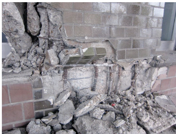
Fig. 7 Column X_1-Y_1 at 1st floor with concrete crushing and rebar buckling
