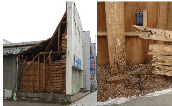
Fig.3 Partial collapse of wooden house in Kurihara
