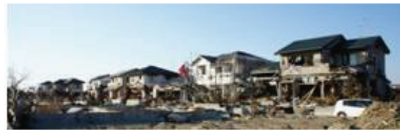
Fig. 25 Wooden houses remained in a line
