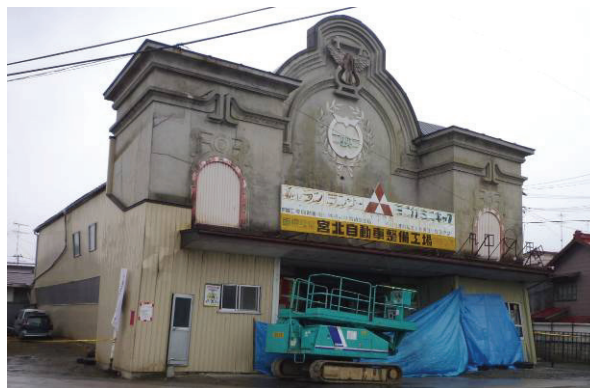
Fig. 18 Severe damage of old cinema in Kurihara-city
