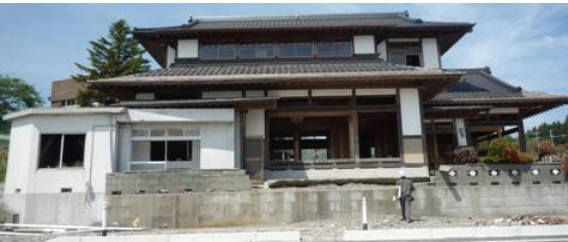
Fig. 45 Traditional wooden house that avoided being carried away under 5-6 m wave depth
