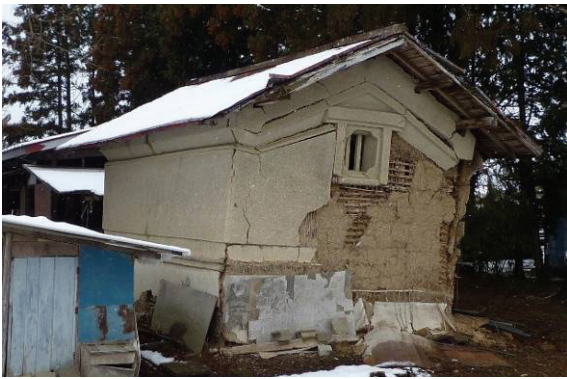
Fig.7 Permanent inclination of a storehouse
