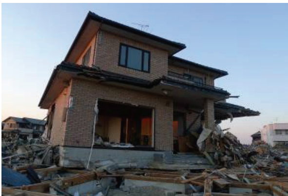
Fig. 28 Wooden house that was carried away with foundation
