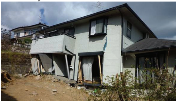
Fig. 21 Severe damage of a house due to landslide in Sendai-city
