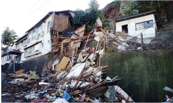
Fig. 19 Collapse of hotel due to landslide in Sendai-city
