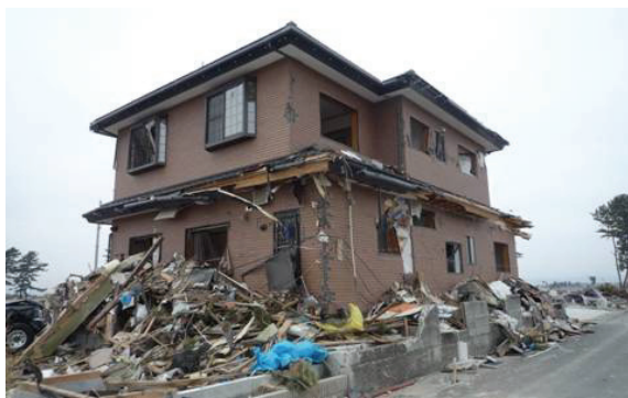
Fig.31 Japanese conventional post and beam wood house remaining (Location (11))
