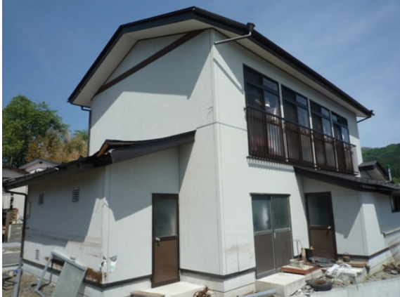
Fig. 44 Wood house without damage with over 7m wave depth
