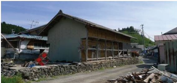
Fig. 48 Warehouse that survived with minor structural specifications
