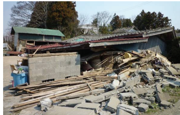
Fig.13 Collapse of shed in Kurihara
