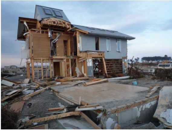
Fig. 36 A portion of a wood house that was washed away
