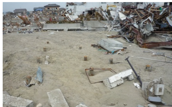
Fig. 29 Steel pile left at the original position of Figure 28
