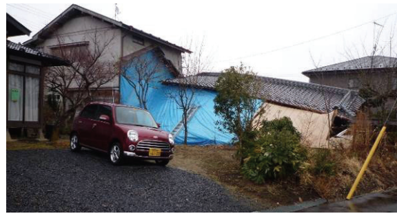
Fig.3 Partial collapse of wooden house in Kurihara
