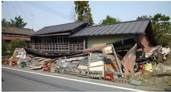
Fig.4 Collapse of wooden house with store attached in Misato
