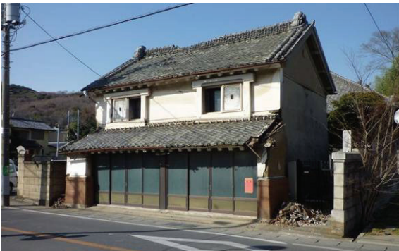
Fig.10 Damage of storehouse with heavy mud walls in Tsukuba
