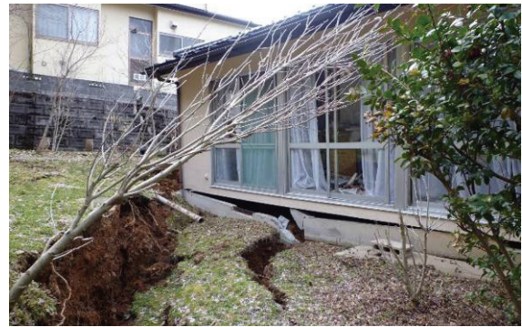
Fig. 20 Severe of a house due to landslide in Sendai-city
