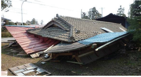
Fig.2 Collapse of wooden house in Osaki
