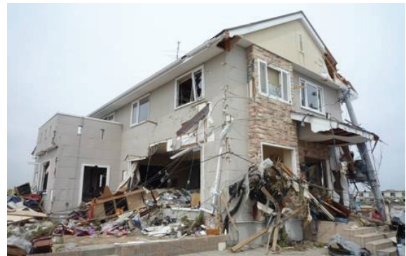
Fig. 32 One of few light frame construction wood houses remaining (Location (11))
