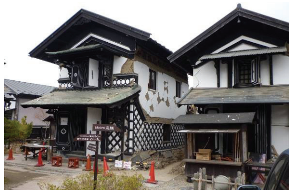
Fig.8 Damage of older storehouses in Osaki
