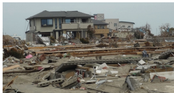
Fig. 34 Wooden houses which avoided being carried away downstream of the factory building (Location (11))
