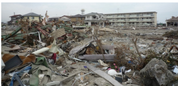
Fig. 33 Group of wooden houses that escaped damage downstream of a RC structure (Location (14))
