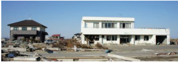
Fig. 24 Wood house remained downstream of RC building
