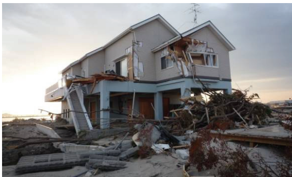
Fig. 38 Hybrid construction consisting of RC on the 1st floor and wooden construction on the second floor
