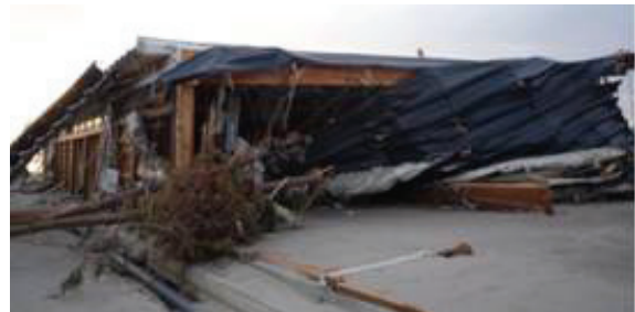
Fig. 39 Heavy timber structure with Glulam frame remaining
