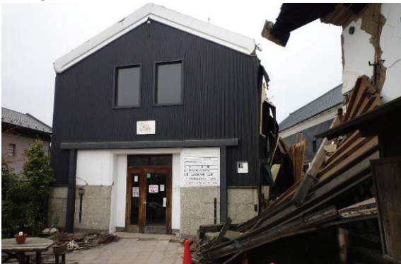
Fig.7 Permanent inclination of a storehouse
