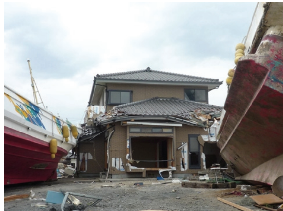
Fig. 41 Wooden house remaining even after collision with ship
