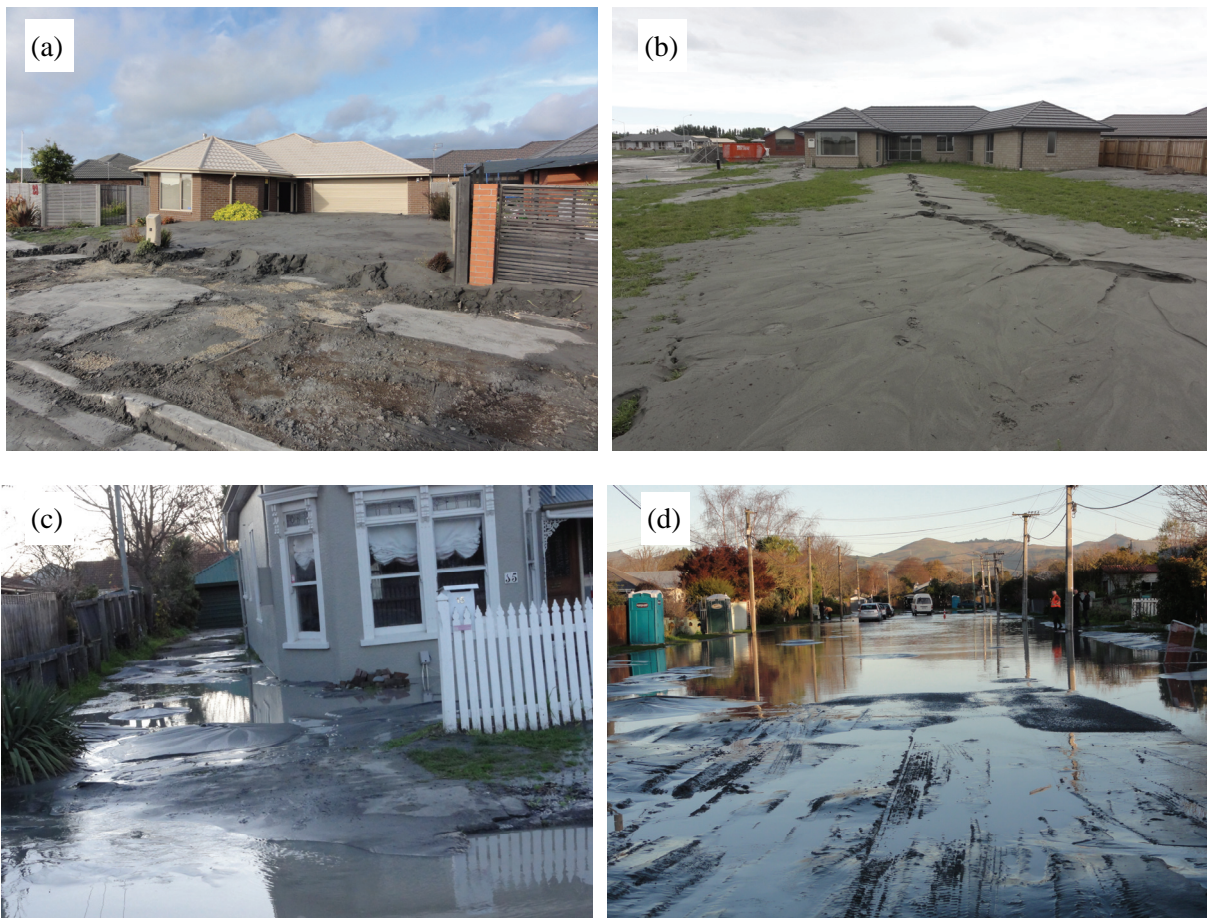
Fig. 6 Severe liquefaction in residential areas (suburbs along Avon River in the abandoned “red zone”)
