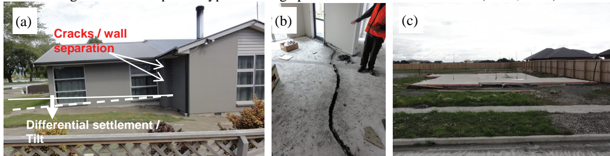
Fig. 8 Schematic plot of typical damage patterns for house foundations (DBH, 2011)
