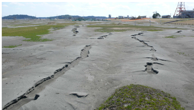
Fig. 3 Silty sand liquefaction at Katori City near Tone River during the Great East Japan Earthquake, Chiba, Japan.
