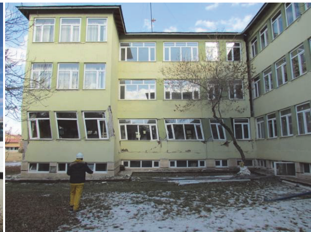
Photo 9 South side of Building C
