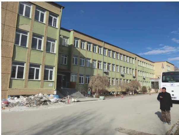
Photo 8 South-east side of the building
