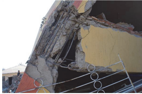
(a) Separation between beam and column (b) Anchorage failure of beam main rebar Photo 5 Details of damaged beam-column joint
