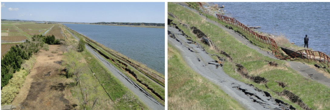
Fig. 6 Views of Hinuma River Levee Slumped and Cracked Due to Liquefaction (GEER 2011b,d)
