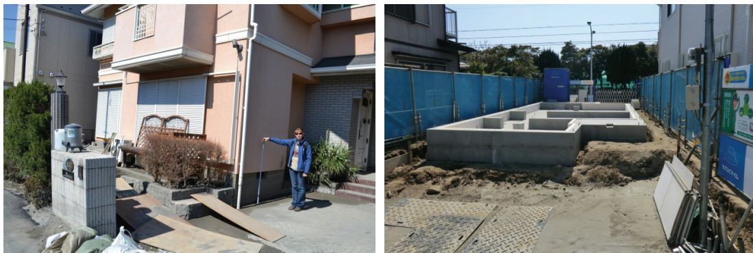
Fig. 3 Tilt and settlement of a residential home in Urayasu (left photo) and a foundation for a residential home in construction (right photo) (GEER 2011)
