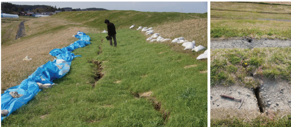
Fig. 7 View of Treated and Untreated Levee Reaches along Naruse River Right Levee at River Kilometer 15.0 - 14.7 (previously treated section in the distance; left photo). Transverse Crack at Boundary between Treated and Untreated Levee Reaches (right photo) (GEER 2011b,d)
