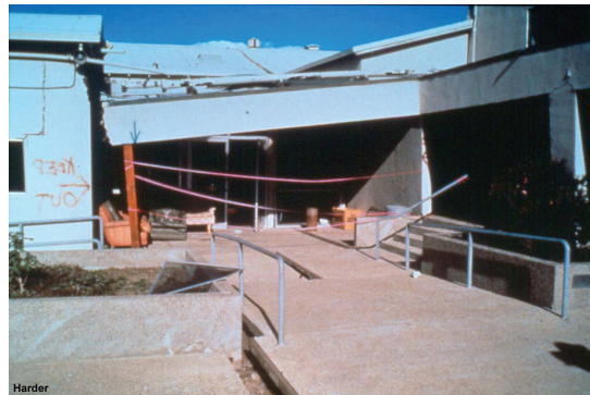
Fig. 4 Wood frame structure on shallow foundations nearly collapsed due to liquefaction-induced stretching of foundation by about 1.3 m in Loma Prieta earthquake (courtesy of L. F. Harder, Jr.)
