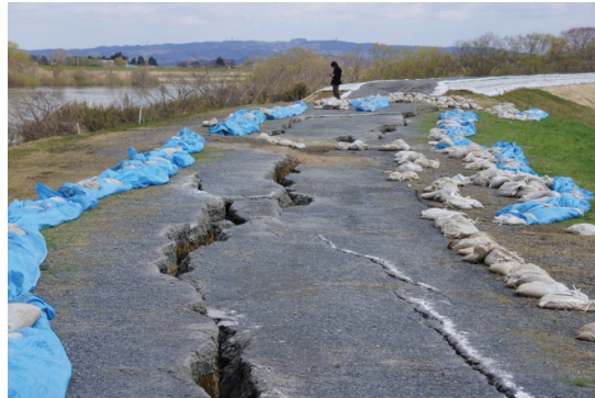
Fig. 5 Levee Damage along Naruse River Left Levee at River Kilometer 11.3 (GEER 2011b,d)
