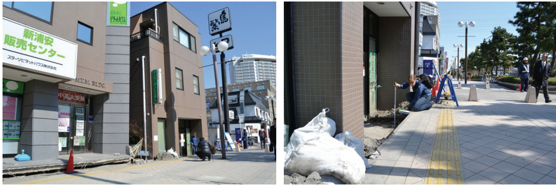
Fig. 2 Differential settlements between a building on piles (gray building on the left), a building on a shallow foundation (brown building on the right), and the ground surface in Urayasu (GEER 2011)
