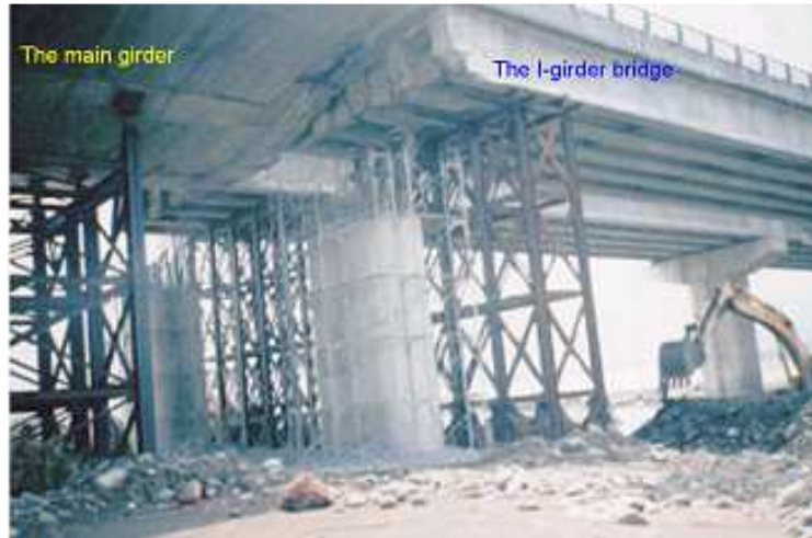
Fig. 7 New cap beam reconstruction
