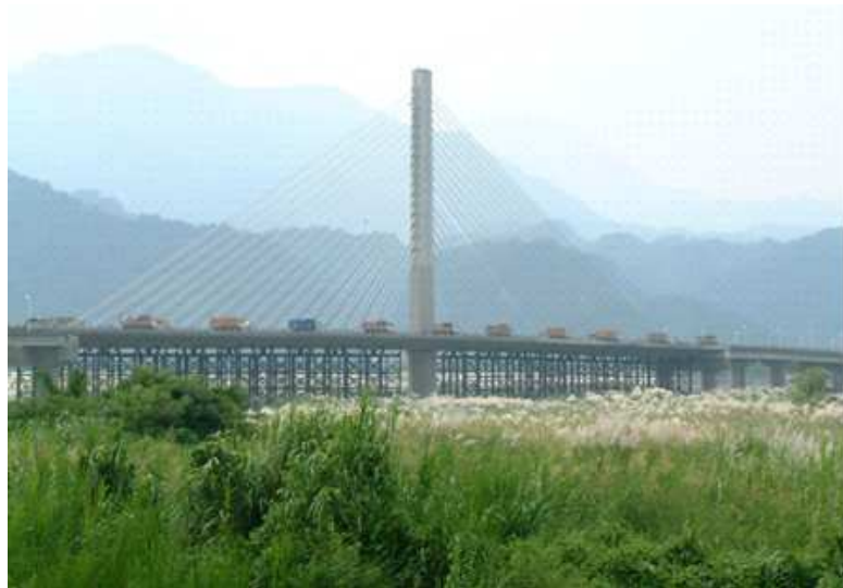
Fig.9 The 1 st loading test after Repair Stage 1
