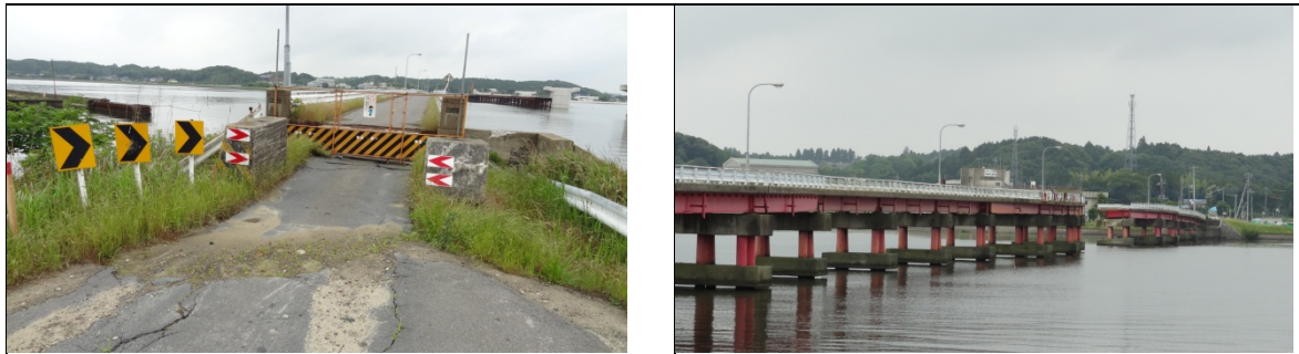
Fig. 13 Damage to Rokko Bridge in Ibaraki Prefecture
