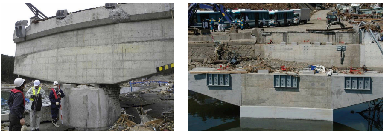
Fig. 11 Broken brackets and restrainers on Utatsu Hashi and Yokozu Kyo Bridges (NILIM, 2011)
