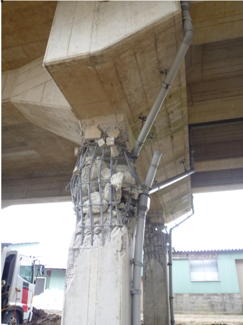
Fig. 17 Damage to Shinkansen Viaducts in Hanamaki
