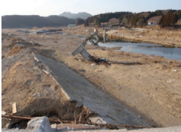
Fig. 9 Damage to JR Kesen-Numa Bridge just upstream from the Koizumi Bridge (Kawashima, 2011)
