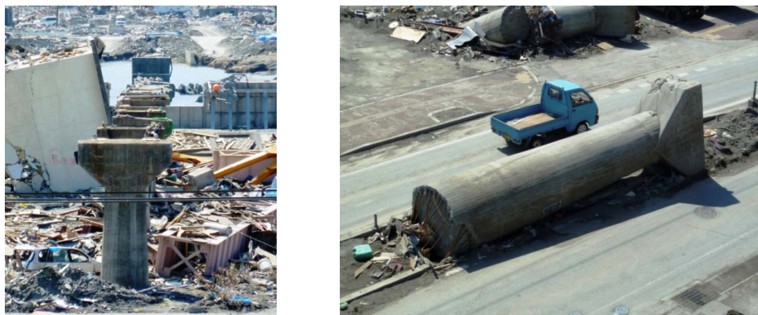
Fig. 5 Undamaged and damaged columns on railway bridge in Otsuchi (Robertson, 2011)
