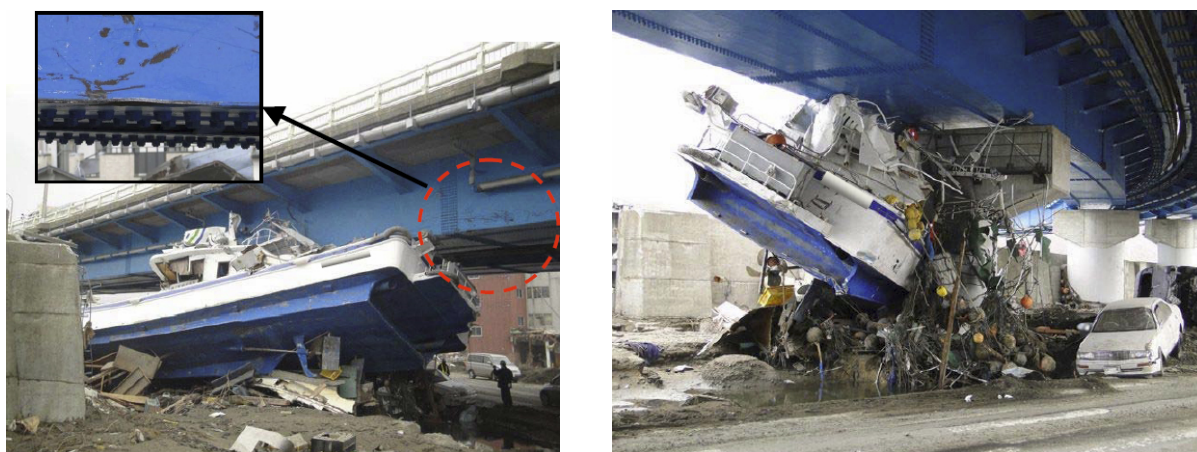
Fig. 4 During the tsunami several boats struck the Miyako Bridge (NILIM, 2011)
