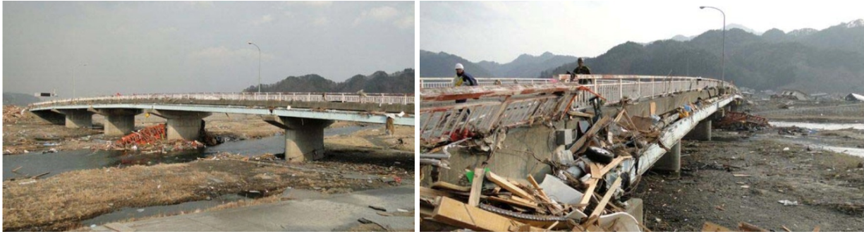
Fig. 6 Bridge across river in Ohamawatari was covered with debris but undamaged (NILIM, 2011)
