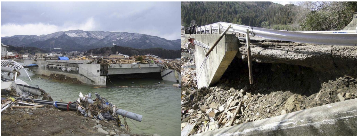
Fig. 7 Embankment scour at Kawaharagawa and Katagishi Bridges along Route 45 (NILIM, 2011)
