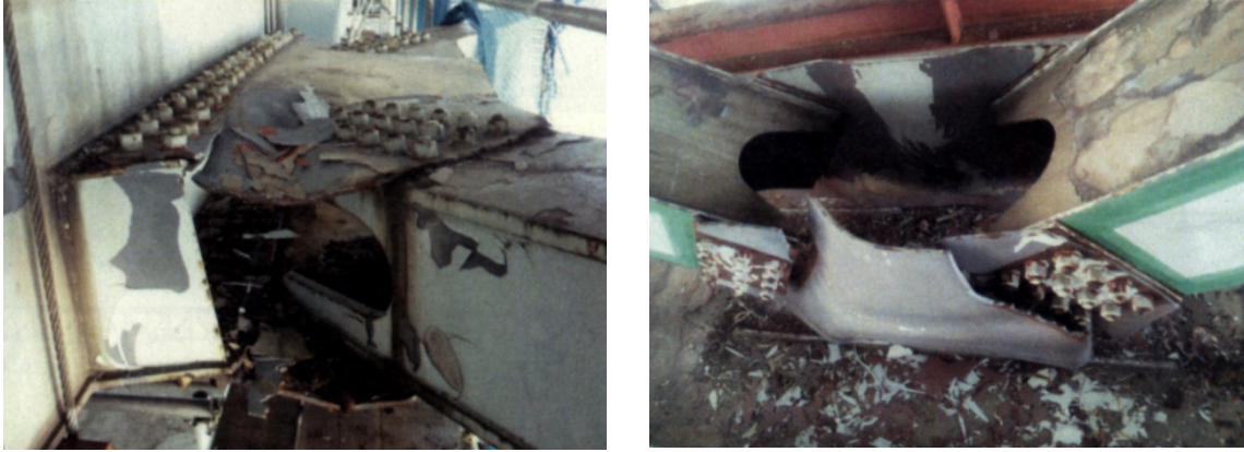
Fig. 15 Gusset plate damage for horizontal and vertical members
