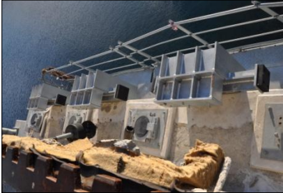
Figure 4. Photo of Utatsu Bridge pier cap between decks B (intact) and C (failed), showing intact unseating prevention devices (UPD's).
