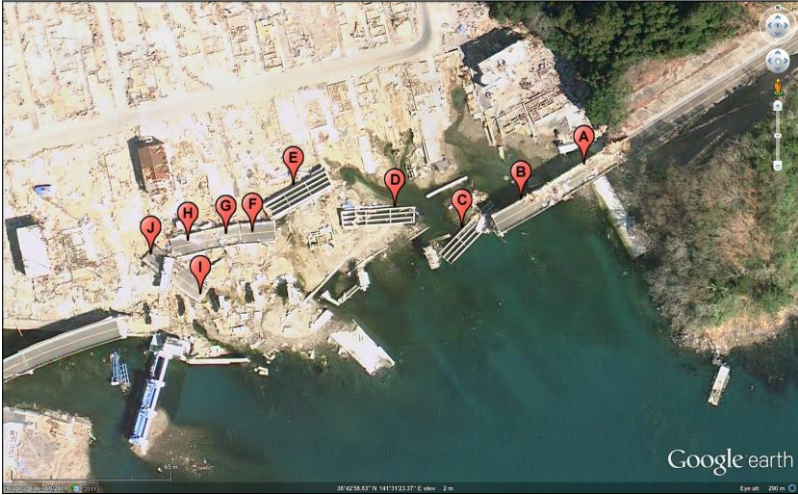
Figure 2. Google Earth image of the Utatsu Bridge on April 6, 2011. Place-marks enumerate individual deck segments.
