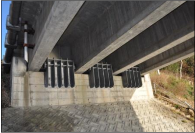
Figure 3. Photo of Utatsu Bridge east abutment (east end of deck A) showing steel and concrete unseating prevention devices (UPD's).
