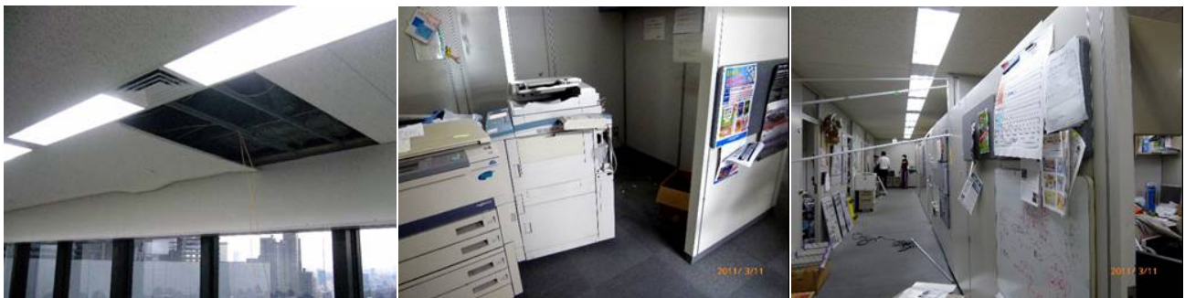
(a) Fall of ceiling panels (b) Movement of a copy machine (c) Deformation of a partition wall
