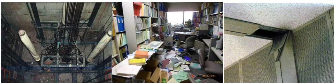
(d) Tangled elevator cable (e) Fall of unsettled objects (f) Fall of cover of EJ
