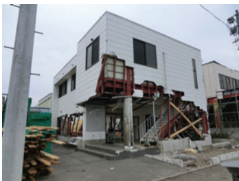
Photo 57 Office building C: external view.
