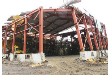
Photo 90 Factory E: cladding washed away.
