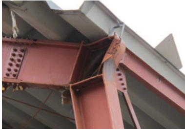
Photo 92 Factory E: large deformation of column panel zone.
