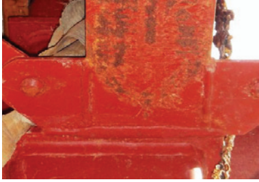
Photo 65 Store A: slight yielding of beam near beam-to-column connection.
