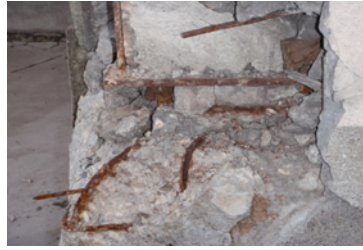
Photo 17 Fracture of anchor bolts, spalling of concrete covering a column base (Miyagino, Sendai)
