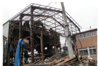
Photo 82 Factory C: external view.
