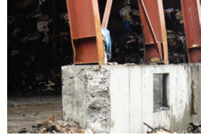
Photo 91 Factory E: local flange buckling of column near base.
