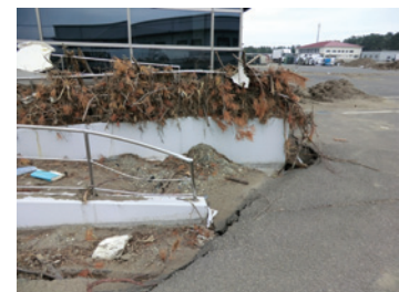
Photo 113 Subsided corner of same building shown in Photo 112 (Iwanuma)
