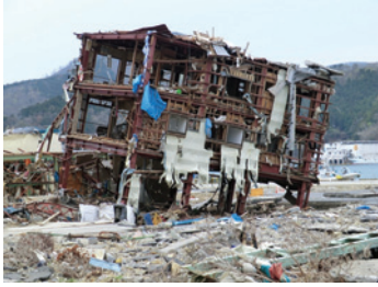
Photo 40 Building A: external view showing large tilt.
