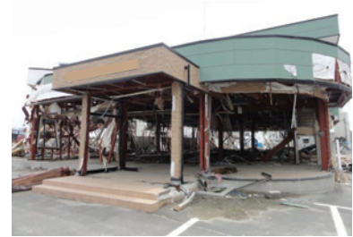
Photo 73 Store B: external view.
