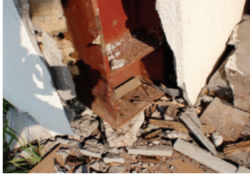
Photo 16 Fracture of anchor bolts (Miyagino, Sendai)
