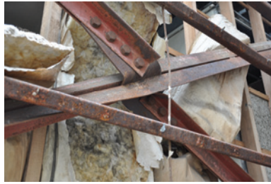
Photo 5 Bending of middle gusset plate in an X-brace (Miyagino, Sendai)
