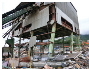
Photo 110 Factory H: first story leaning towards inland.
