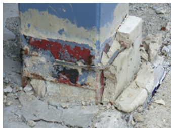
Photo 14 Spalling of concrete covering a column base (Koriyama)
