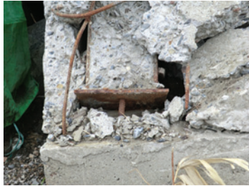
Photo 101 Factory F: damage to concrete encasing column base.
