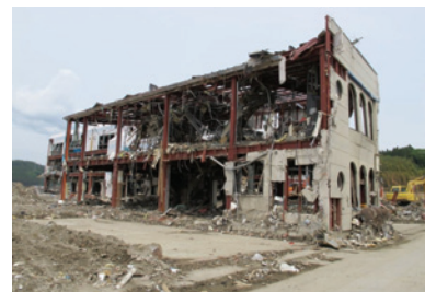
Photo 88 Store E: damage to cladding.
