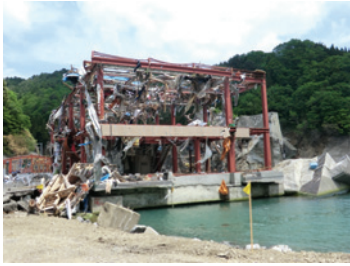
Photo 107 Office building F: exterior view.
