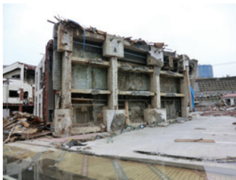
Photo 43 Building B: view of foundation showing fracture piles.
