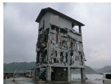
Photo 106 Ice making factory A: exterior view.
