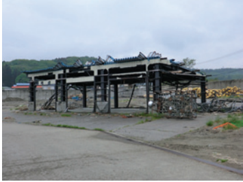
Photo 98 Warehouse D: nonstructural elements washed away.
