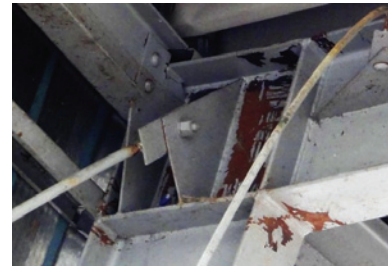
Photo 85 Factory D: yielding of joint region.
