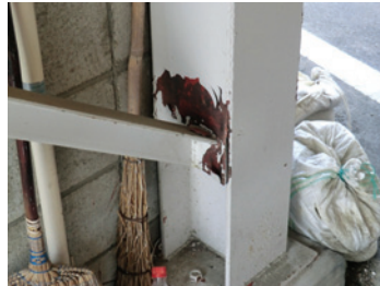
Photo 8 Yielding of column web near bracing connection (Koriyama)
