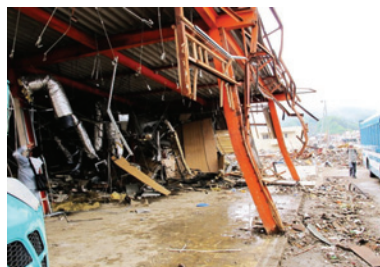
Photo 78 Store C: distorted columns.
