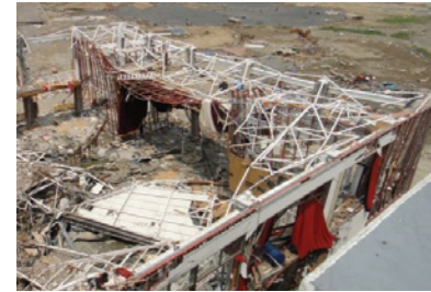
Photo 70 Elementary school gymnasium A: severely damaged roof.
