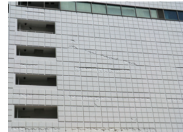
Photo 24 Cracking of external finish (Aoba, Sendai)
