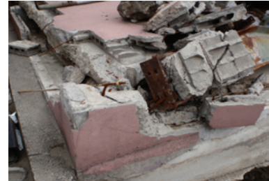
Photo 39 Port facility B: fractured anchor bolt.
