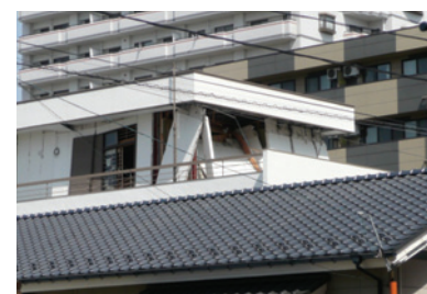
Photo 27 Fallen and twisted cladding (Koriyama)
