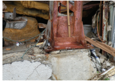
Photo 53 Warehouse A: damage to column base.
