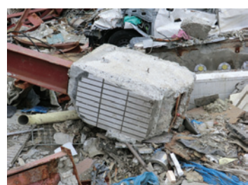
Photo 51 Building E: column base.
