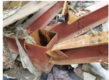
Photo 45 Building C: failed connection.
