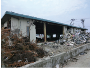
Photo 31 Office building A: External view.
