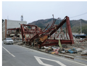
Photo 44 Building C: external view.
