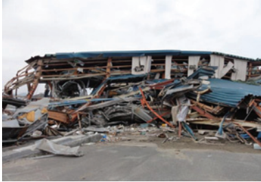
Photo 71 Warehouse C: external view.
