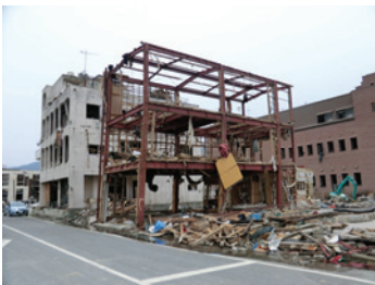
Photo 46 Building D: external view.
