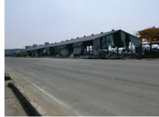
Photo 35 Port facility A: external view.
