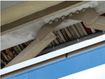
Photo 7 Out-of-plane deformation of gusset plate (Miyagino, Sendai)
