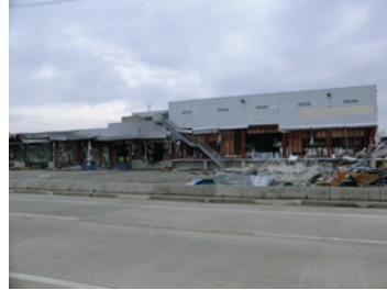
Photo 102 Factory G: external view.
