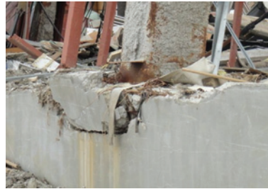
Photo 69 Elementary school gymnasium A: damaged column base.
