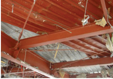
Photo 89 Store E: deformed metal floor slab.
