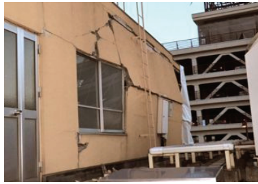
Photo 29 Damaged cladding in a mechanical penthouse (Koriyama)
