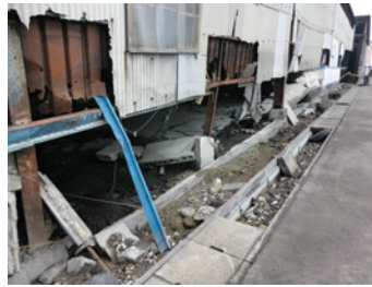
Photo 56 Warehouse B: view of front side; far-right end subsided.
