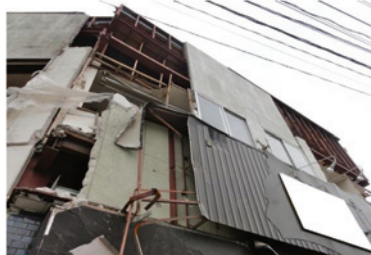
Photo 26 Fallen cladding (Ishinomaki)
