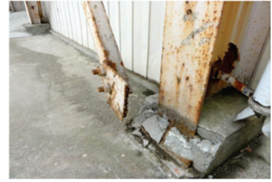
Photo 6 Fracture of gusset plate-to-column weld and spalling of concrete covering an exposed base plate (Ishinomaki)
