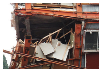
Photo 76 Traditional hotel A: close-up view of collapsed second story.
