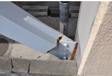
Photo 10 Out-of-plane deformation of gusset plate caused by compression (Miyagino, Sendai)
