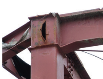
Photo 50 Building E: beam-to-column connection.
