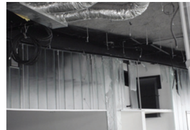
Photo 21 Fallen ceiling, partitions damaged by impact (Aoba, Sendai)
