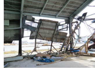
Photo 36 Port facility A: inside view.
