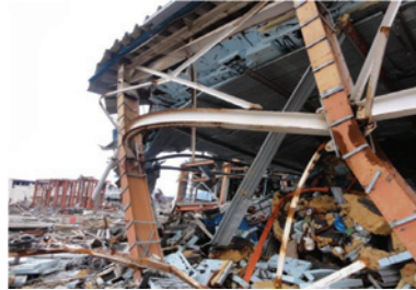
Photo 72 Warehouse C: deformed columns and beams.
