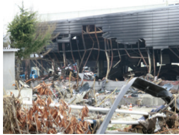
Photo 115 Building (Miyagino, Sendai)
