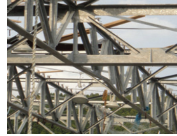
Photo 67 Factory A: buckled chord members in roof truss.
