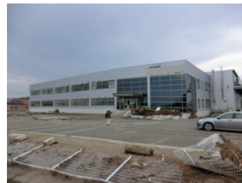
Photo 112 Office building: Two right-end spans subsided due to liquefaction. (Iwanuma)
