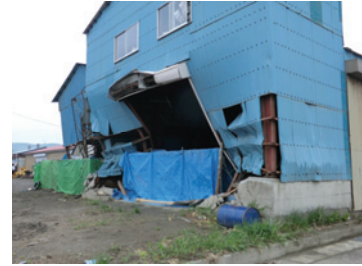
Photo 100 Factory F: cladding remained.
