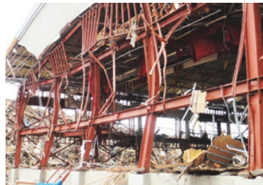
Photo 96 Gymnasium C: severely distorted columns.
