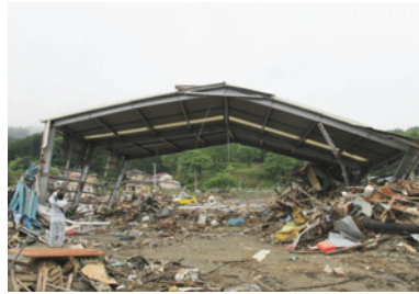
Photo 84 Factory D: building leaning towards right.
