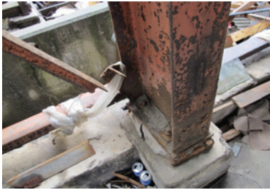
Photo 83 Factory C: net section fracture of a single-angle brace at the column base.
