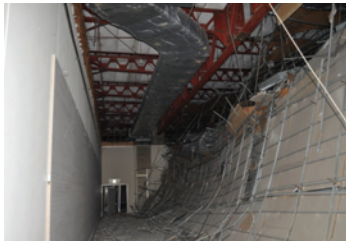
Photo 19 Fallen ceiling grid and boards (Fukushima)
