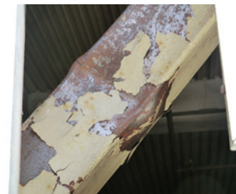
Photo 3 Local buckling in square-HSS brace (Aoba, Sendai)
