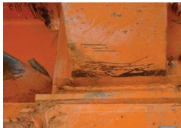
Photo 63 Office building E: yielding of beam near beam-to-column connection.
