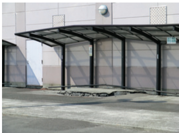
Photo 111 Shopping complex: ground subsided near footing foundation. (Rifu)
