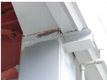
Photo 1 Yielding of an older built-up column (Koriyama)
