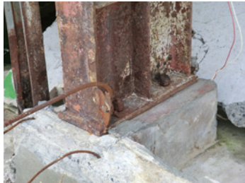
Photo 37 Port facility A: column base rusted presumably due to seawater proximity.
