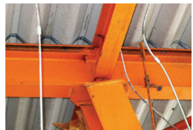
Photo 79 Store C: plastic deformation at top of first-story column.
