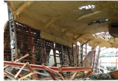
Photo 54 Warehouse A: inside view.
