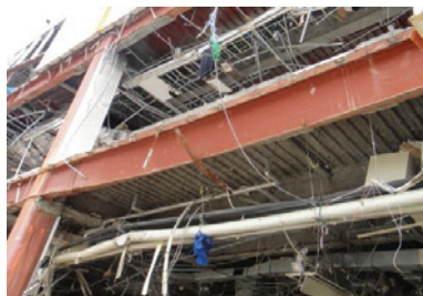
Photo 87 Store D: torsional deformation of beam.
