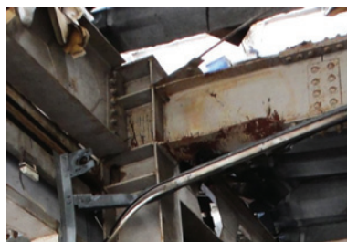
Photo 81 Factory B: yielding in beam-to-column connection.
