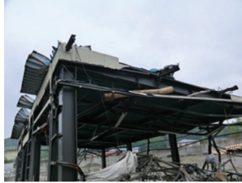
Photo 99 Warehouse D: minimal structural damage; no residual drift.
