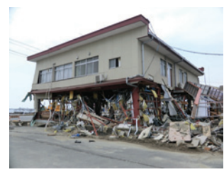
Photo 33 Office building B: external view showing noticeable residual drift.
