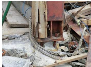
Photo 47 Building D: column base lifted and anchor bolts deformed.
