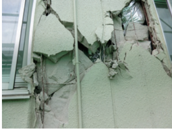
Photo 28 Damage to cladding covering a column (Wakabayashi, Sendai)
