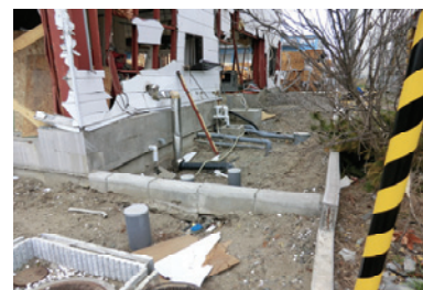
Photo 59 Office building C: under-ground piping exposed after scouring.
