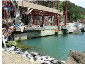
Photo 108 Office building F: foundation exposed after scouring.
