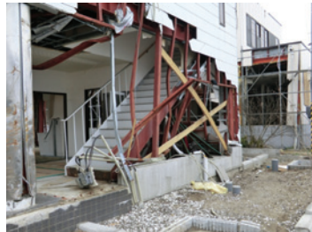
Photo 58 Office building C: severe damage to cladding.
