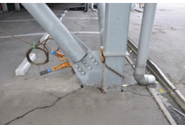
Photo 13 Cracking of asphalt covering a column base (Miyagino, Sendai)
