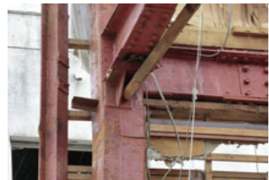
Photo 48 Building D: beam-to-column connections at corner
