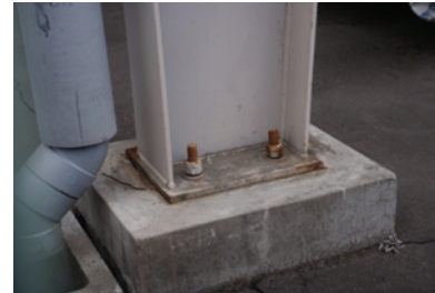
Photo 12 Elongation of anchor bolts in an exposed base plate (Miyagino, Sendai)
