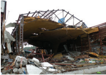
Photo 52 Warehouse A: external view.
