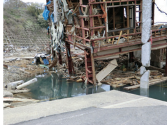
Photo 41 Building A: foundation scour.
