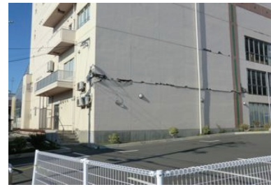
Photo 30 Damaged cladding (Sukagawa)
