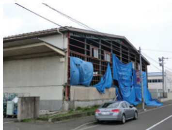
Photo 25 Failure of metal lath-and-mortar cladding (Miyagino, Sendai)
