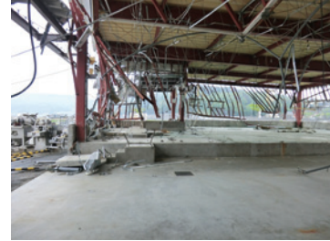
Photo 103 Factory G: little structural damage.
