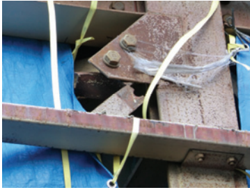
Photo 4 Net section fracture of single-angle brace (Miyagino, Sendai)
