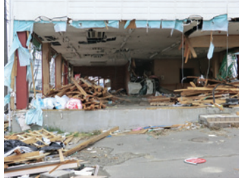
Photo 61 Office building D: nonstructural damage in first story.
