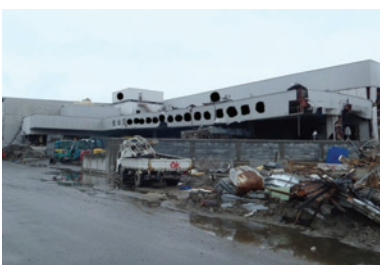
Photo 80 Factory B: external view.
