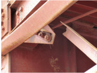
Photo 34 Office building B: net section fracture of a single-angle brace.
