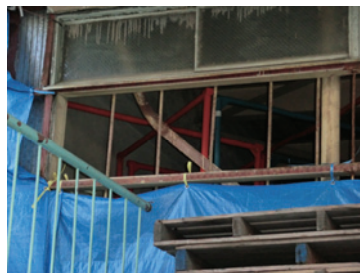
Photo 2 Buckling of double-angle brace (Miyagino, Sendai)
