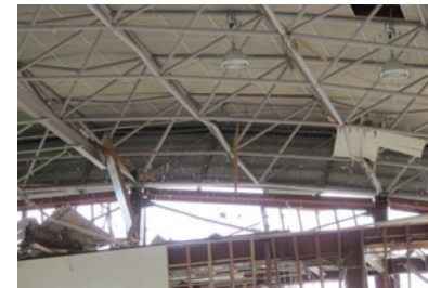
Photo 97 Gymnasium C: distorted roof trusses.
