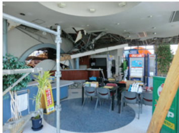
Photo 22 Partly fallen ceiling (Koriyama)
