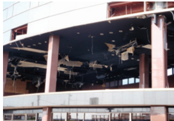
Photo 20 Fallen claddings; damaged ceiling boards (Miyagino, Sendai)
