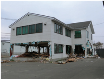
Photo 60 Office building D: cladding washed away in first story; minimal structural damage.
