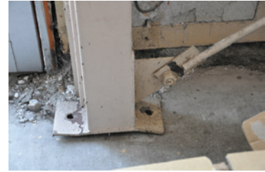
Photo 18 Fracture of anchor bolts, out-of-plane deformation of base plate (Miyagino, Sendai)
