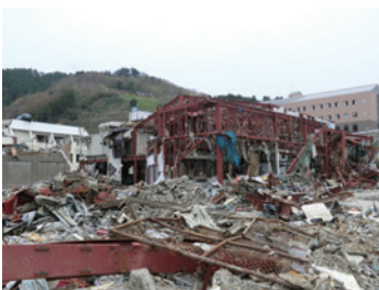
Photo 49 Building E: external view.
