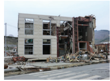
Photo 42 Building B: building collapsed towards left.
