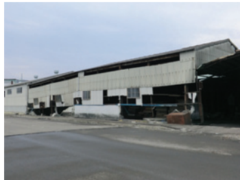
Photo 55 Warehouse B: external view; right end subsided.
