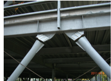
Photo 9 Out-of-plane deformation and fracture of gusset plates (Miyagino, Sendai)
