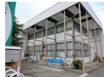
Photo 23 Fallen ceiling on the outside of a building (Wakabayashi, Sendai)
