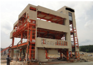
Photo 62 Office building E: majority of nonstructural elements washed away; minor structural damage.
