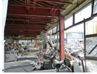
Photo 32 Office building A: inside view.
