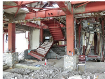
Photo 105 Hotel B: interior damage seen at first story.
