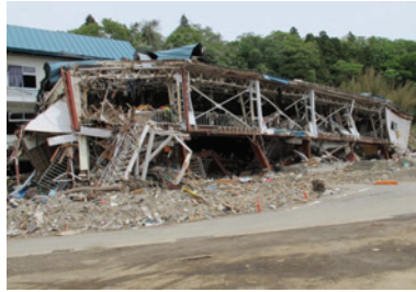
Photo 93 High-school gymnasium B: external view of collapsed building.
