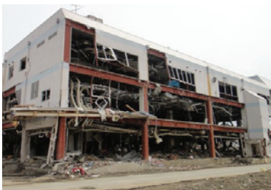
Photo 86 Store D: damage to cladding.
