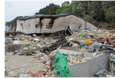
Photo 94 High-school gymnasium B: building displaced by 20 m.
