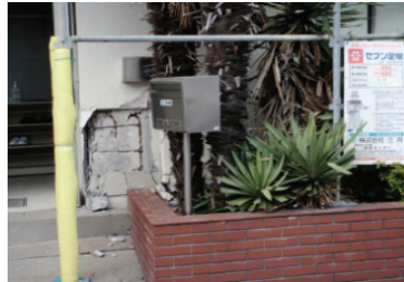
Photo 11 Spalling of reinforced concrete encasing a steel column base (Wakabayashi, Sendai)
