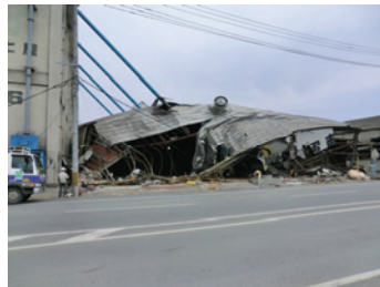
Photo 38 Port facility B: external view.
