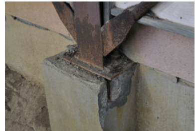
Photo 15 Spalling of reinforced concrete foundation supporting a column base (Koriyama)
