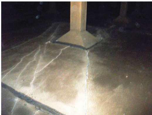
Fig. 1: Huntsbury No.1 Reservoir – base-slab cracking (22 February 2011 damage mapping).
