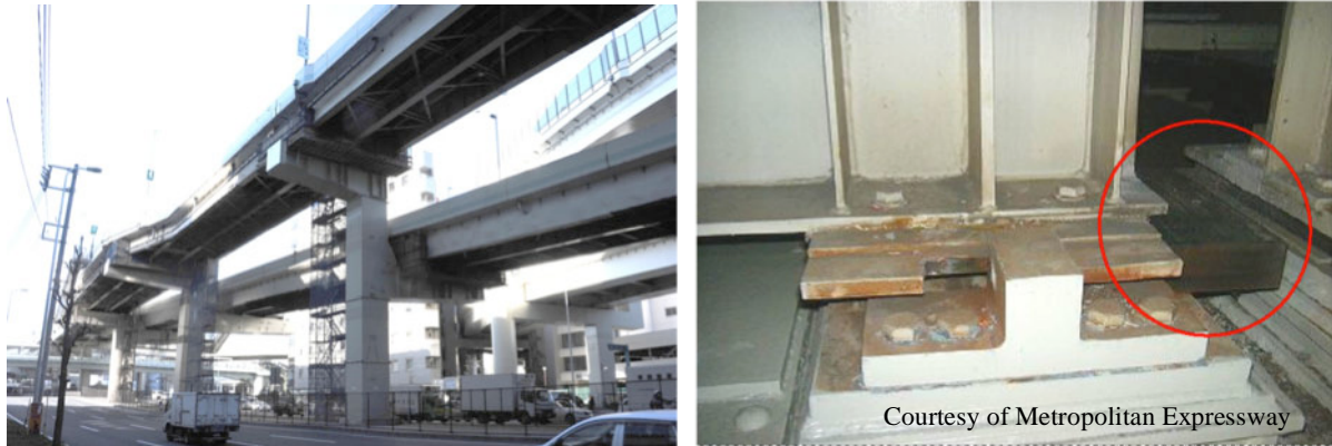
Photo 8 Kinko JCT Viaduct and damage of rubber pad
