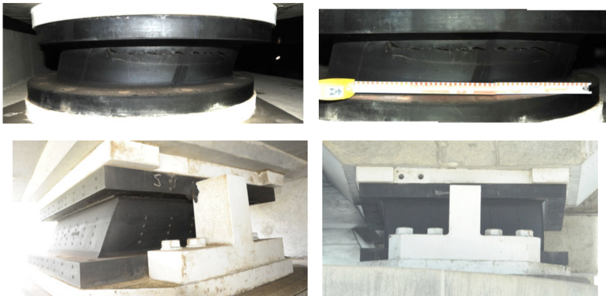
Photo 7 Damage of lead rubber bearings of Asahi Viaduct
