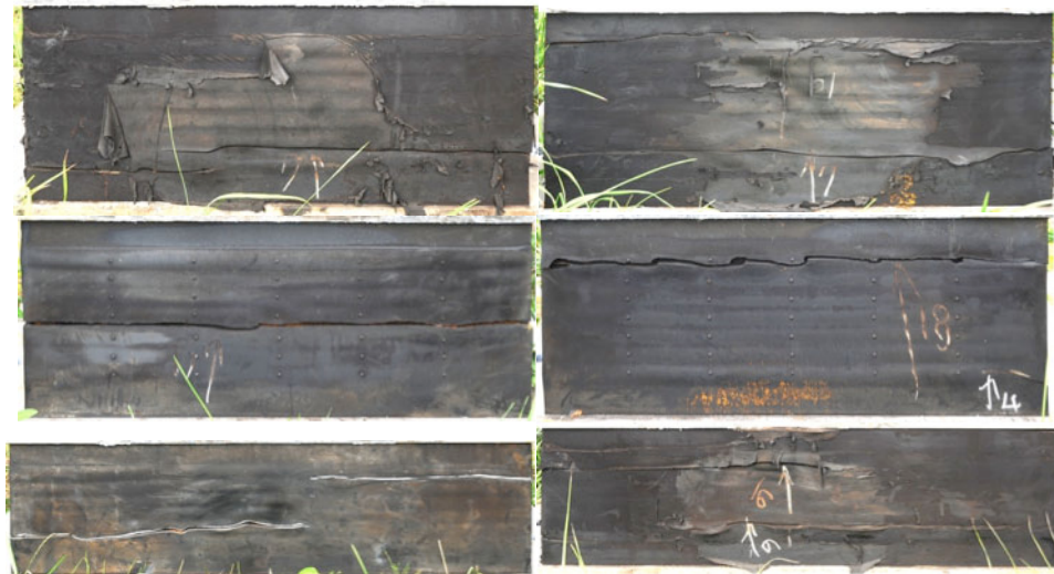
Photo 4 Various crack patterns of damaged elastomeric bearings of Rifu Viaduct
