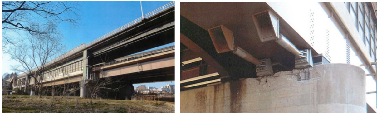
Photo 9 Nakanose bridge and damage of anchors of dampers
