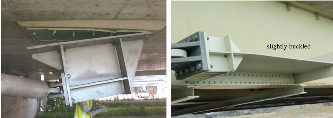
Photo 10 Damage of attachments of dampers in bridges
