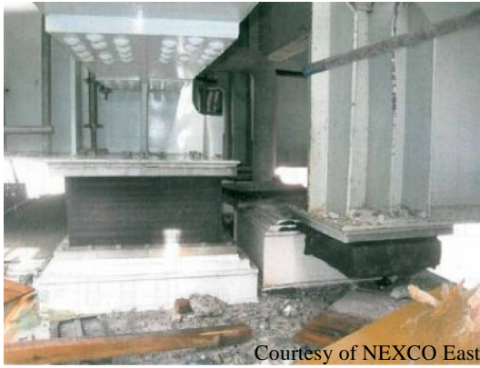
Photo 2 Rupture of elastomeric bearings of Tobu Viaduct
