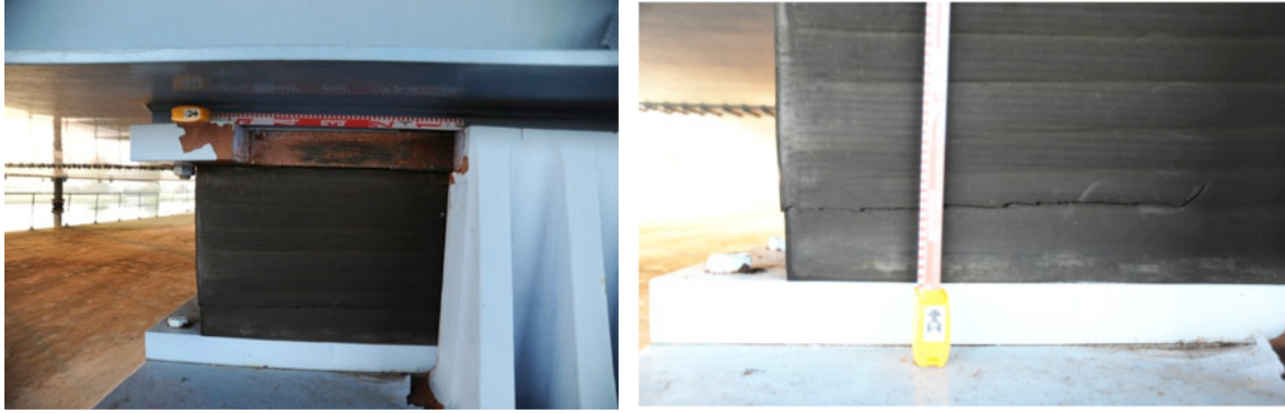
Photo 5 Ruptured elastomeric bearings of Shin Nakagawa Bridge
