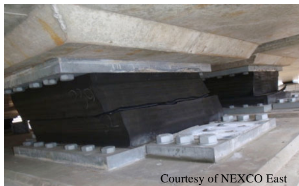
Photo 3 Rifu Viaduct and rupture of elastomeric bearings
