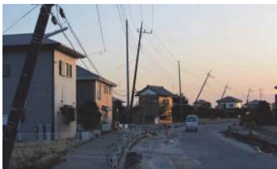
Photo 1 A large volume of sand boil was observed, and many telephone poles became slanted. The telephone pole standing straight was installed after the earthquake. (Hinode, Itako)
