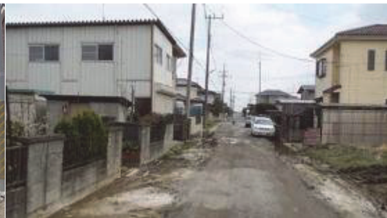
Photo 4 Traces of sand boils spreading on the road (Iwai Greenland, Bando)
