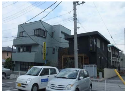
(1) Outside of the tilted house
