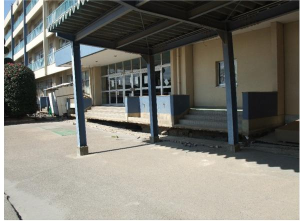
Fig. 5 Post-liquefaction ground settlement at Sawara Junior High School
