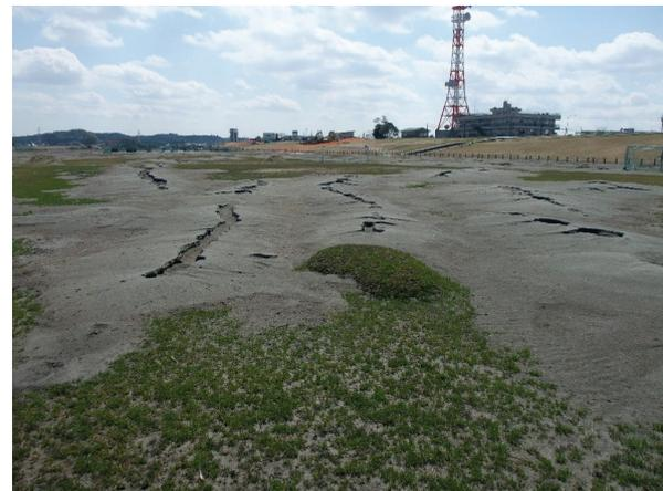
Fig. 7 Sand boils at the dry river bed of Tonegawa River (view towards river embankment)
