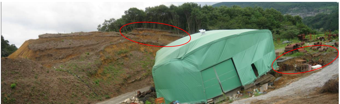
Fig. 10 Huge tension cracks present along the top of the landslide, showing the presence of deep seated slip planes.
