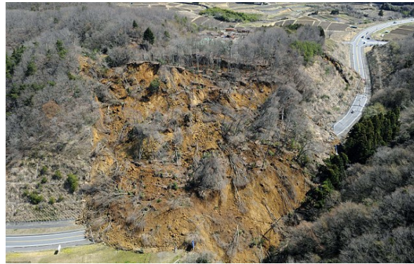
Fig. 4 An aerial view of the landslide mass (Photo by Kyodo News). The coherent landslide mass flushed the road passing by its toe.
