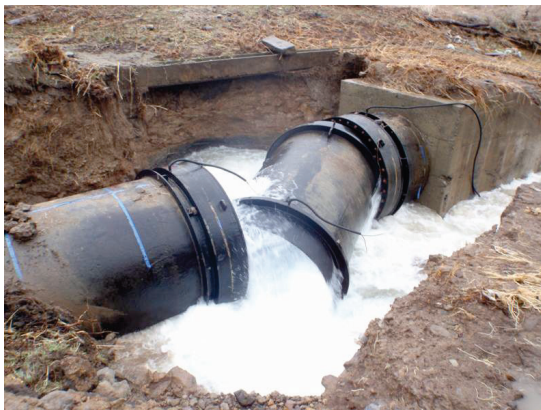
Photo 1 Damage to steel pipe with 2400mm diameter ( Miyagi Pref.) 1) .
