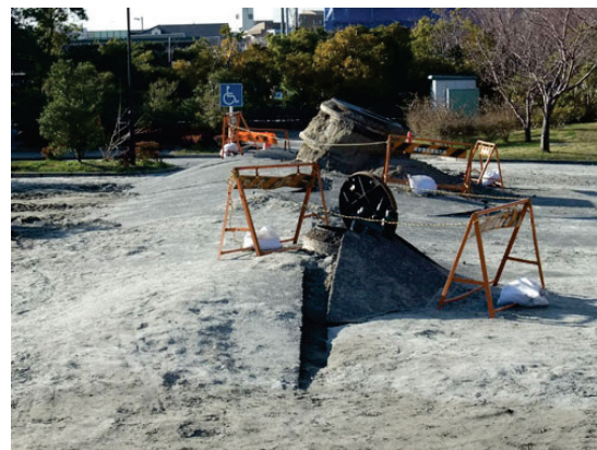
Photo 2 Uplift of underground water tank (Chiba Pref.) 2) .
