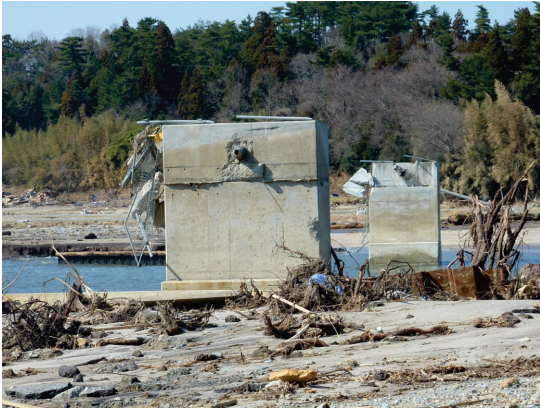
Photo 3 Damage to water pipe bridge (Miyagi Pref.) .
