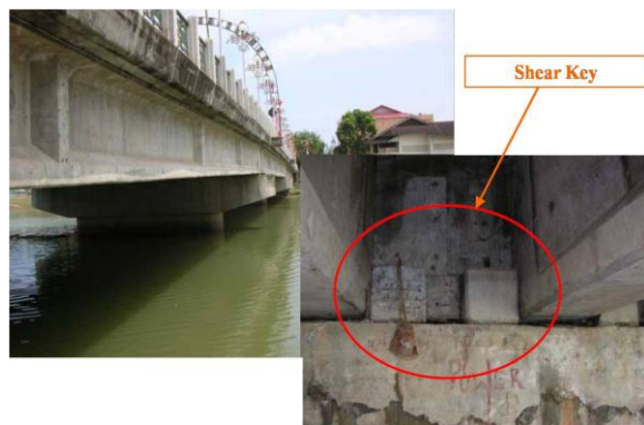
Figure 4 Survived the Concrete Bridge at Banda Aceh in Indonesia (2004)
