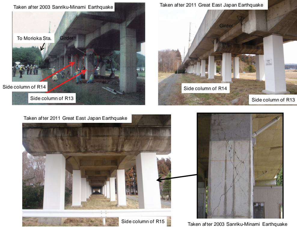
Figure 4. R13 to R15 of the No. 5 Inohana viaduct taken after the 2003 Sanriku-Minami earthquake and the 2011 Great East Japan earthquake (Note: the viaducts were retrofitted before the 2011 Great East Japan earthquake)
