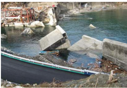
(a) Seawalls toppled due to scouring at Miyako city
