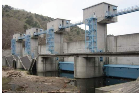
(c) Tsunami flew over the tsunami wall across Fudai River (TP+15.5m), and broke maintenance decks / main structure stayed intact at Fudai village
