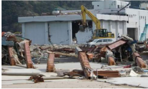
(a) Bent steel pillars at Onagawa town
