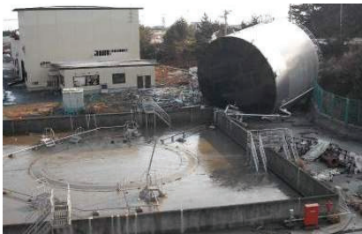
(c) Fuel tank floated and dislocated (Tohoku EPCO) at Onagawa town
