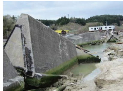
(b) Seawalls toppled due to scouring at Miyako city
