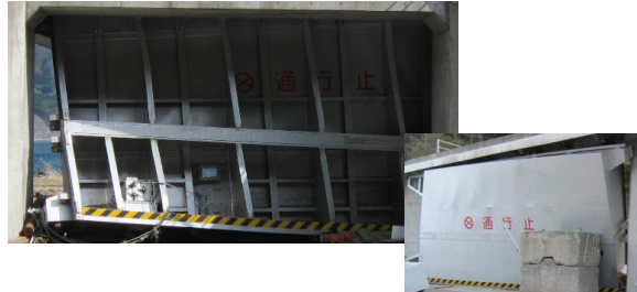
(b) Sea wall gate destroyed by impulsive tsunami force at Miyako city
