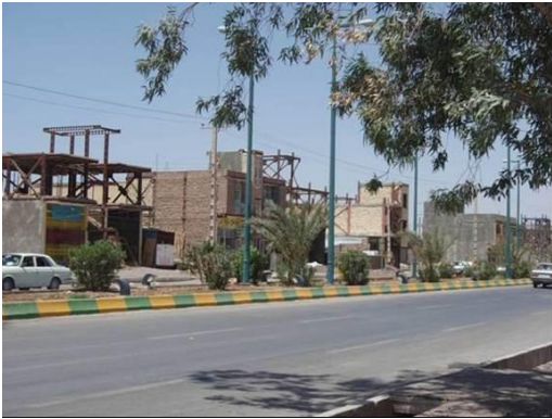
Photo 3: Bam, Iran after 2003, reconstruction
