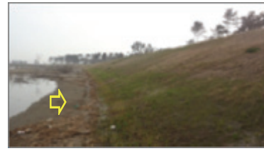
Photo 2 Front slope on May 2
