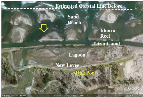
Photo 1 Around new river levee on April 6
