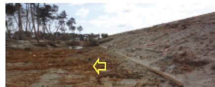
Photo 4 Back slope and toe on May 2
