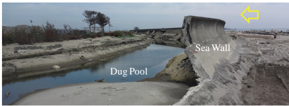
Photo 12 Dug pool at sea wall on June 9
