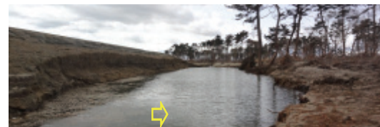
Photo 5 Slight slope failure on May 2
