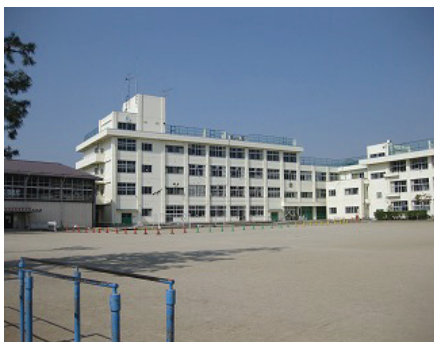
Fig. 23. North view of building
