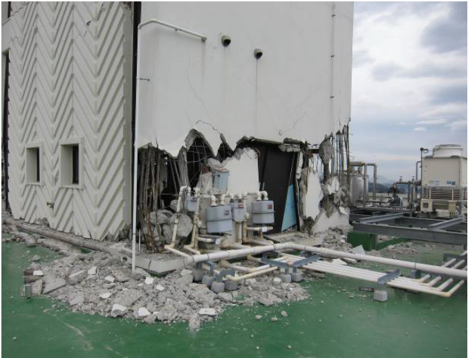
Fig. 18 Collapse of penthouse
