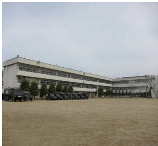
Fig. 9 Overall view of damaged school building
