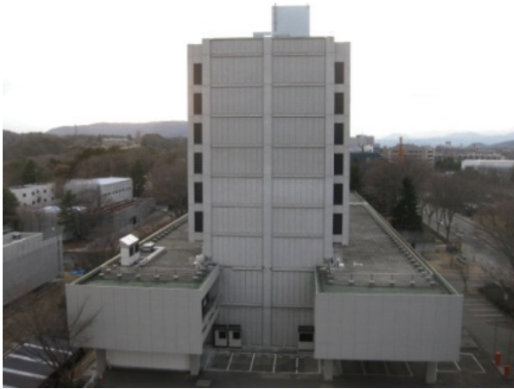
Fig. 12 Civil Engineering Building in Tohoku Univ.
