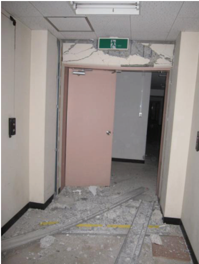
Fig 17. Shear failure in short beams
