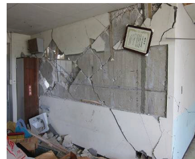
Fig. 11 Shear failure in shear wall
