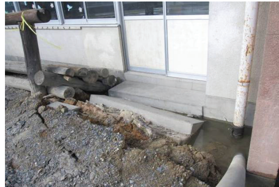
Fig. 29 Liquefaction evidence located 3 stair steps from the ground surface.
