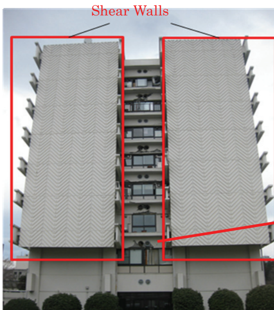
(a) Coupled shear wall and link beam
