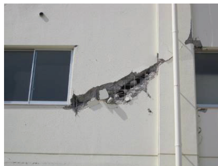
Fig. 24 Shear failure in wing wall
