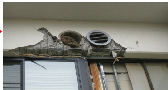
(b) Close up of shear failed coupling beam
