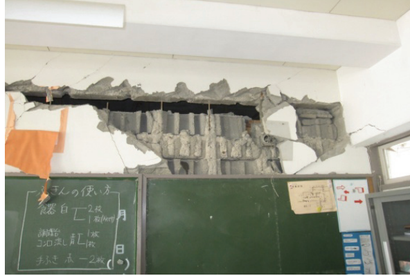
Fig. 27 Partial collapse of concrete blocks partition wall
