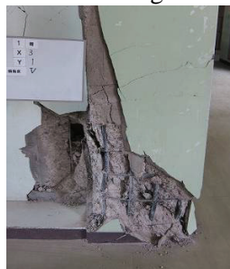
Fig. 10 Shear failure in column
