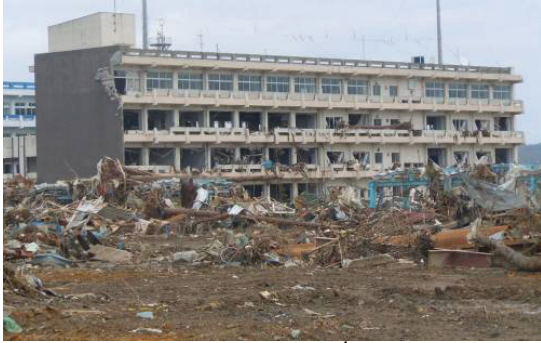
Fig. 30 Flood reached 3 rd floor
