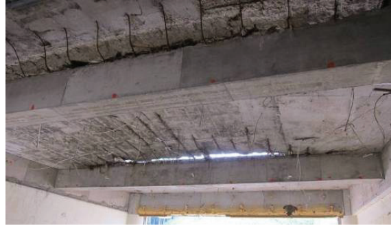
Fig. 31 Slab uplifted and dismantled from beam
