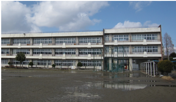
Fig. 28 Settlement of school building in Osaki City
