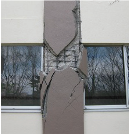
Fig.20 Shear failure in column
