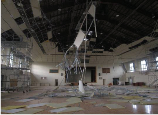
Fig. 26 Large parts of the false ceiling fell down
