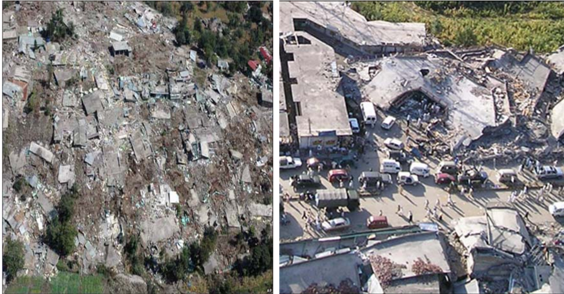
Fig. 2 Devastation caused by Kashmir Earthquake in Muzaffarabad and Balakot cities
