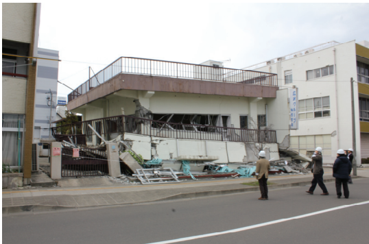
Photo 2: Reinforced concrete building destroyed by the earthquake. (Sendai city)
