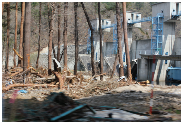
Photo 14: Sluice gates (village side). The tsunami exceeded the height of the gates slightly, so some trees have been knocked down, but the wave did not reach the residential area and so human casualties were avoided. (Fudai village)
