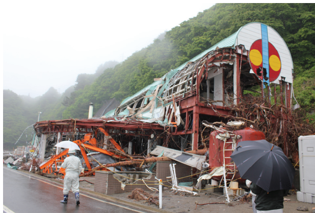
Photo 19: Steel frame structure of aquarium near oil reserve facility. Only the skeleton remains. On the day of the disaster, all visitors were able to retreat to safety thanks to advance warnings. (Kuji city)
