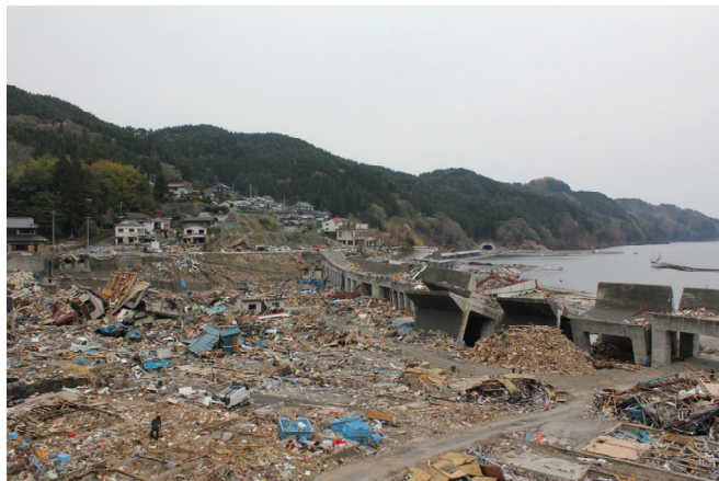
Photo 15: Fallen seawalls by the tsunami and destroyed town. There is a person who is standing in dumb surprise in the lower left. (Kamaishi city, Touni town)
