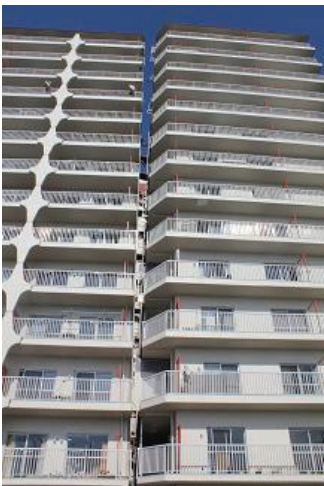
Photo 3: Leaning high-rise residential building. (Sendai city)
