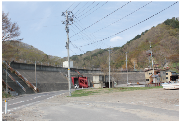
Photo 11: 15.5m high seawall. The houses behind the wall remain undamaged. Photo taken from the sea side of the wall. (Fudai village)
