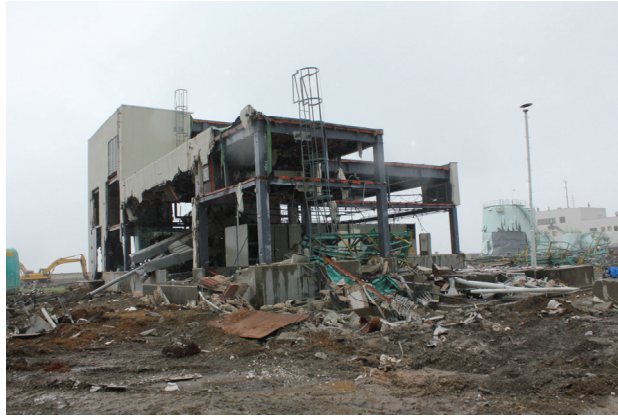
Photo 18: Steel frame structure at national oil reserve facility. The site, excavated from a mountainside, escaped damage (Kuji city)
