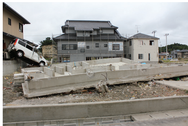
Photo 22: A mat foundation flown by the tsunami from another place to here. A northern part in the prefecture.
