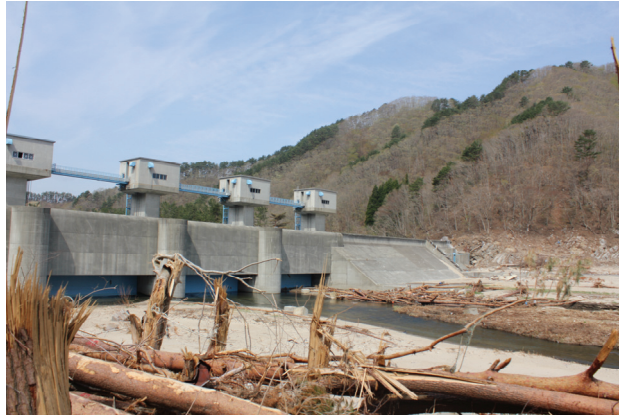
Photo 13: Sluice gates (sea side). Trees have been knocked down in the foreground. (Fudai village)
