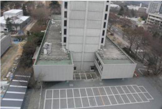
Photo 1: Building damage at Tohoku University (esp. 3rd floor column base)
