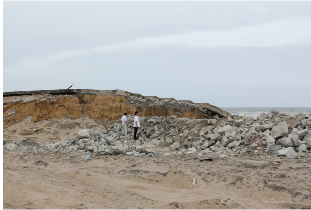
Photo 21: Broken breakwater by the tsunami that is located very close to Fukushima Prefecture (the right). The Pacific Ocean is visible (the right).
