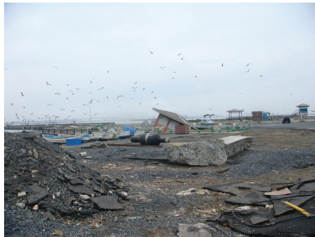
Photo 17: Area around Kabushima, Port of Hachinohe, Aomori prefecture. The force of the tsunami has tilted the reinforced concrete toilet building in the centre of the image.
