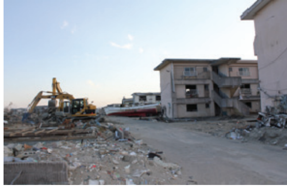
Photo 4: Tsunami-damaged reinforced concrete apartment building. Wooden houses were washed away, and only the foundations remain. (Natori city)
