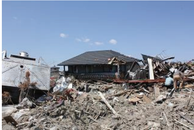
Photo 7: Washed away and destroyed homes. A mound of rubble has been formed in the foreground. (Ishinomaki city)
