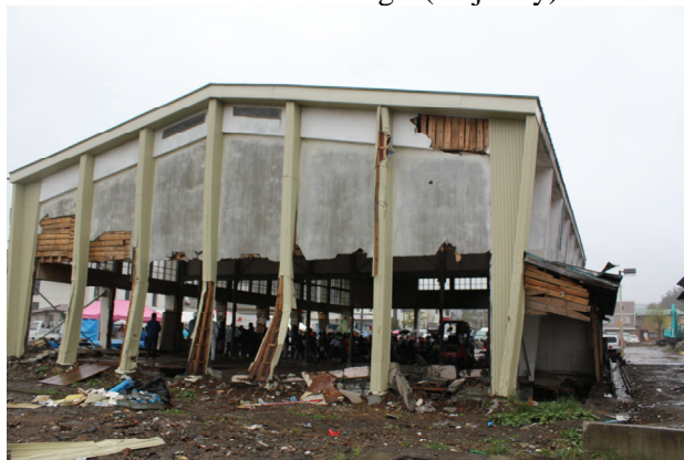
Photo 19: Steel frame structure of aquarium near oil reserve facility. Only the skeleton remains. On the day of the disaster, all visitors were able to retreat to safety thanks to advance warnings. (Kuji city)
