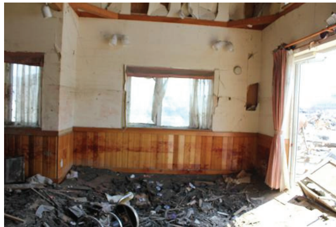
Photo 8: Interior of a house destroyed by the tsunami. The floor has been swept away by water pressure. Taken with consent. (Ishinomaki city)
