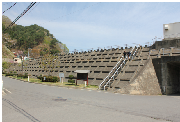
Photo 12: The 15.5m seawall from the previous photo, photographed from the opposite (village) side. Compare size with the two people on the steps. (Fudai village)
