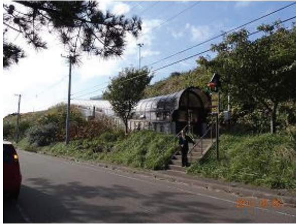
Photo 24: Covered evacuation route to high ground. (Aonae area)
