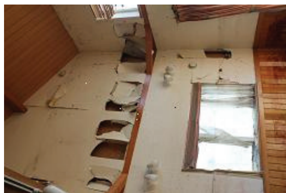
Photo 9: Interior of a house destroyed by the tsunami. Water pressure has made holes in the wall. Taken with consent. Same house of the Photo 8. (Ishinomaki city)
