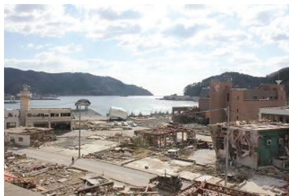
Photo 6: Overturned reinforced concrete structure and damage to coastal structure. The aforementioned cylindrical tank (Photo 5) is seen on its side. (Onagawa town)
