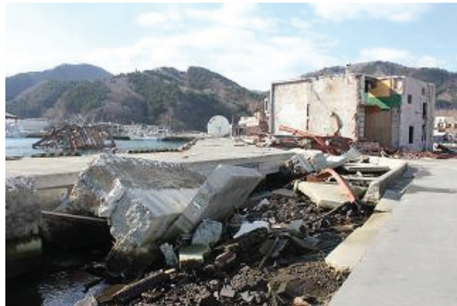
Photo 5: Overturned reinforced concrete structure and damage to coastal structure. A cylindrical tank is visible in the distance. (Onagawa town)
