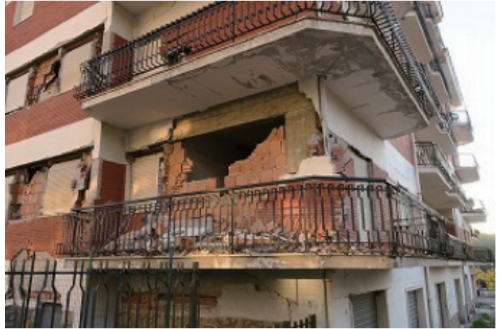
Damage of infilled brick wall (Amatrice)
