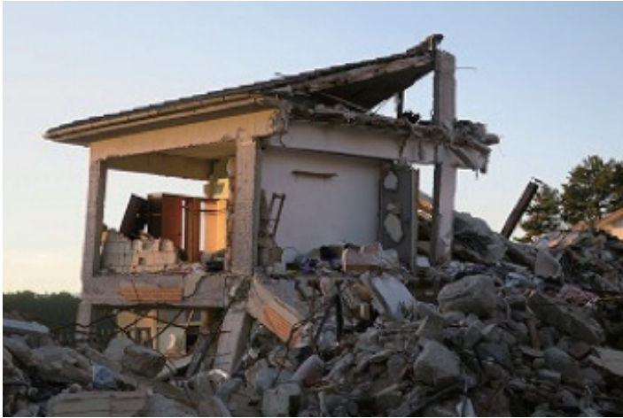
Damage of RC joint (Amatrice)
