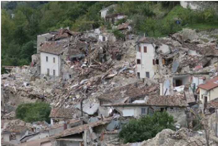
Damage of masonry buildings (Pescara del Tronto)
