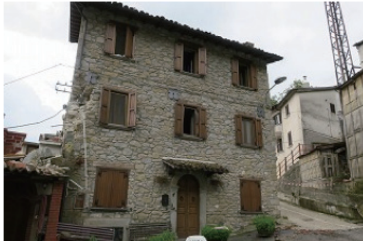
Masonry building with tie bar (Pescara del Tronto)
